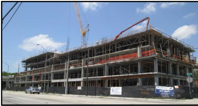
Site construction - May 2014
