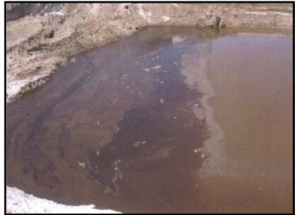
Free floating product in excavation
