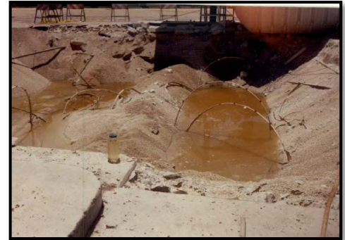
Tank removal excavation (1991)
