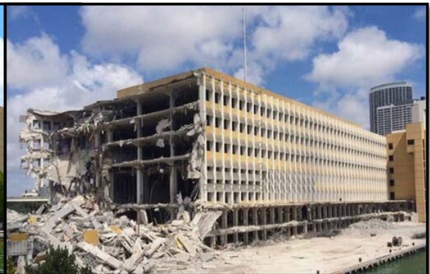
Demolition of Miami Herald Building (2014)
