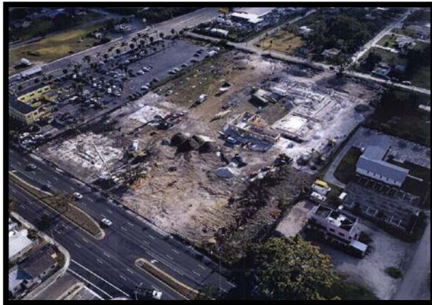
Prior to site construction (April 13, 2006)
