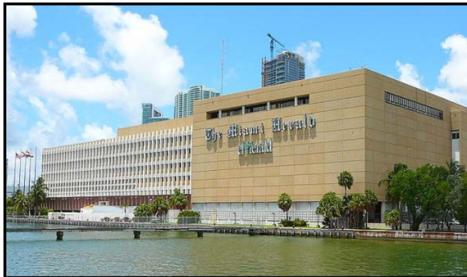
Former Miami Herald Building
