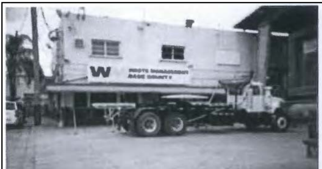
Former Waste Management Facility
