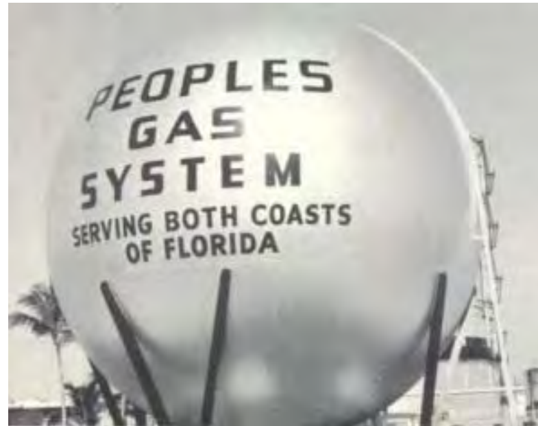
Peoples Gas Storage Tank-Miami-Florida (Date Unknown)
