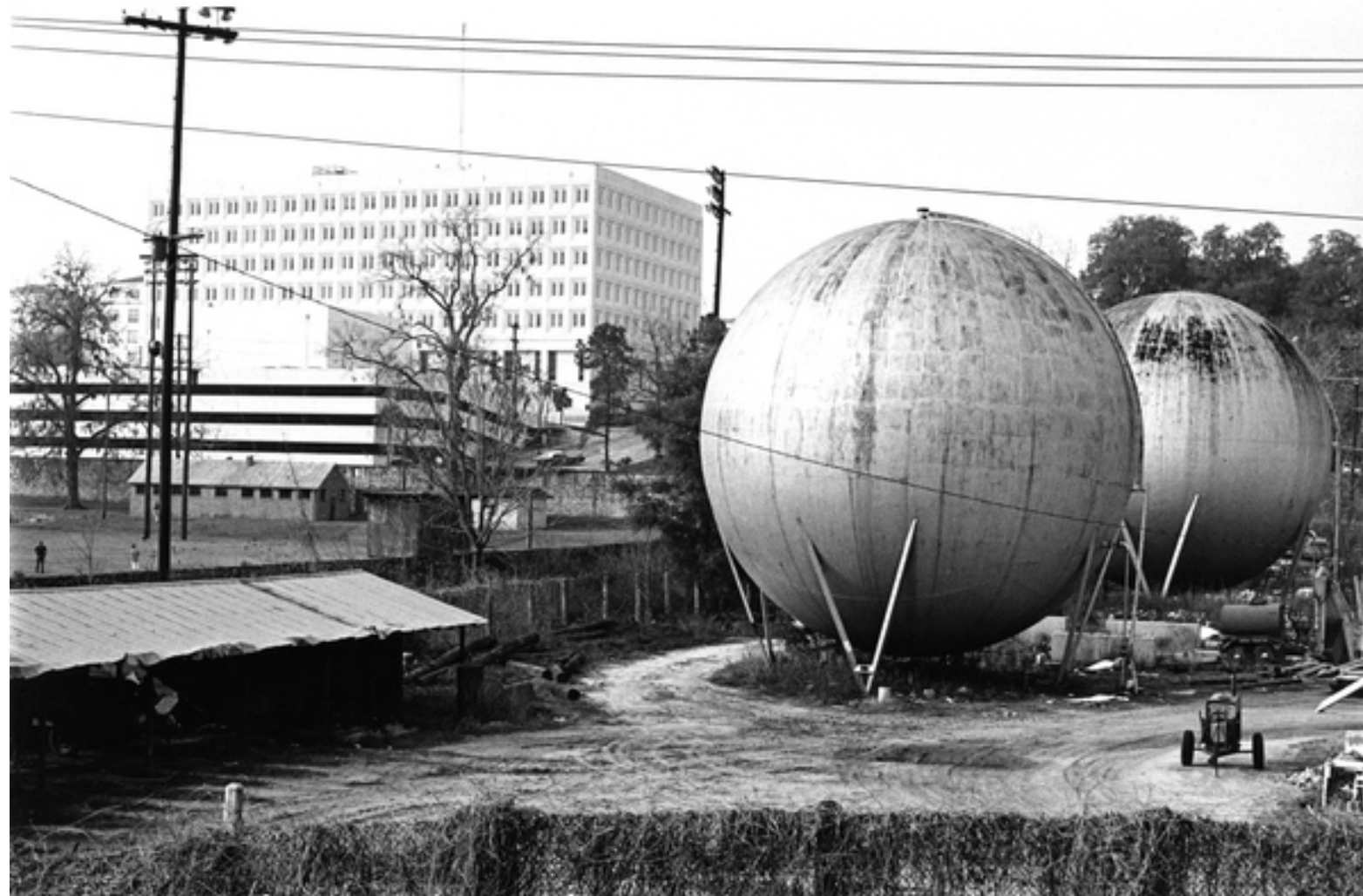
City of Tallahassee MGP (aka: Cascade Park Gasification Plant) Hortonspheres/Gas Holders, Centennial Field to Left (Date Unknown)
