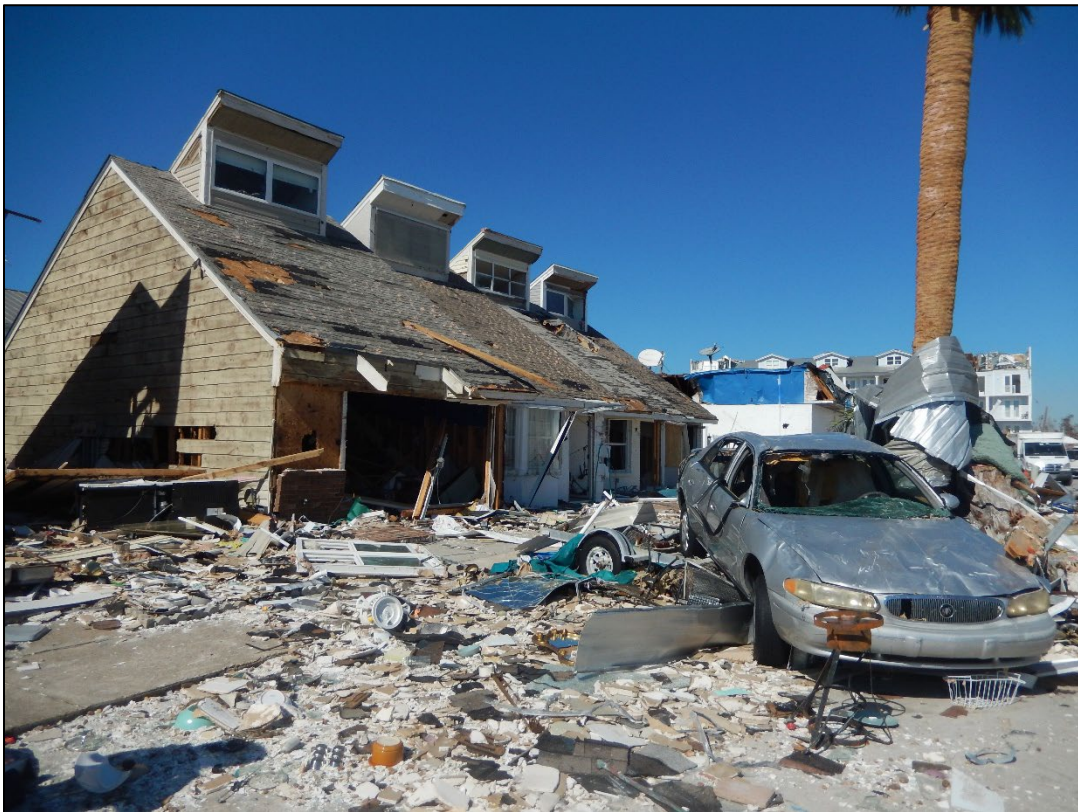
Figure 31. Multifamily dwelling destroyed near R129, Mexico Beach.
