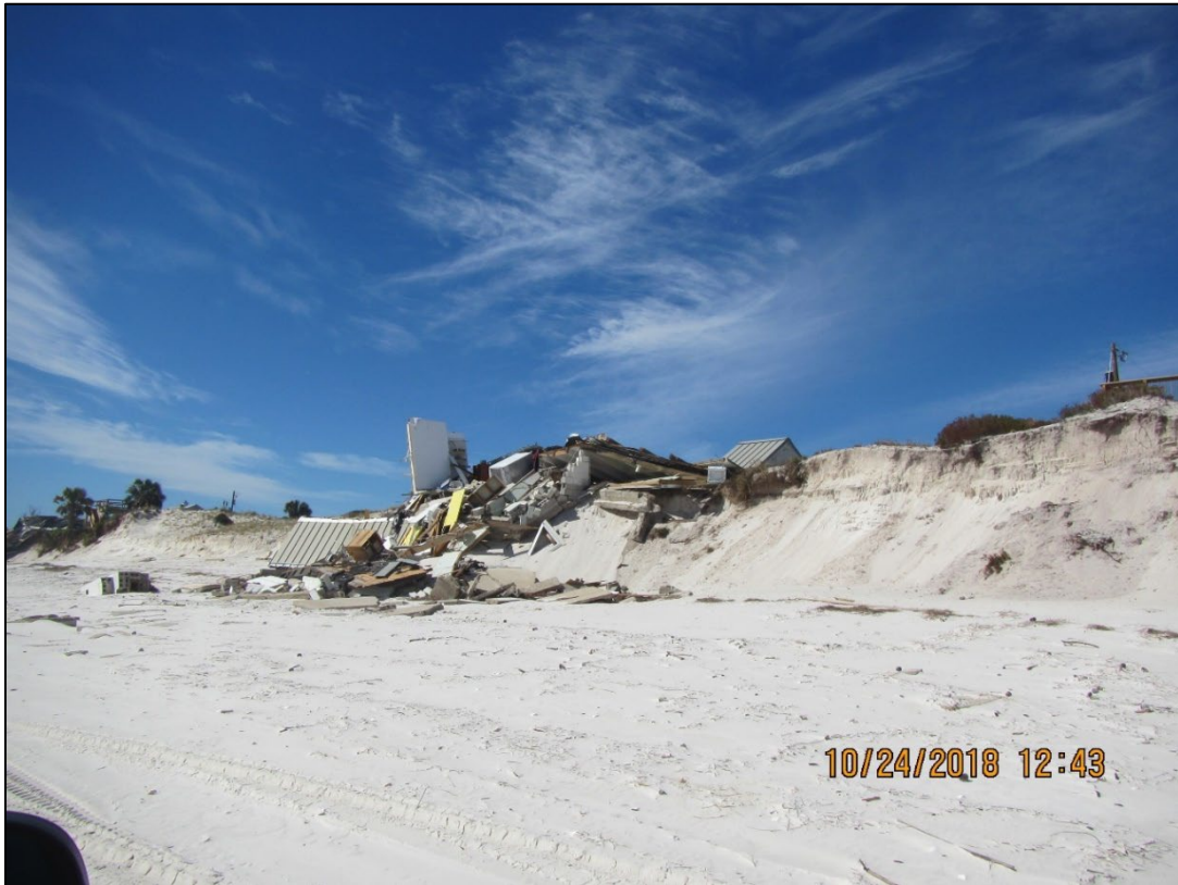
Figure 95. Dwelling destroyed near R176, Dog Island.
