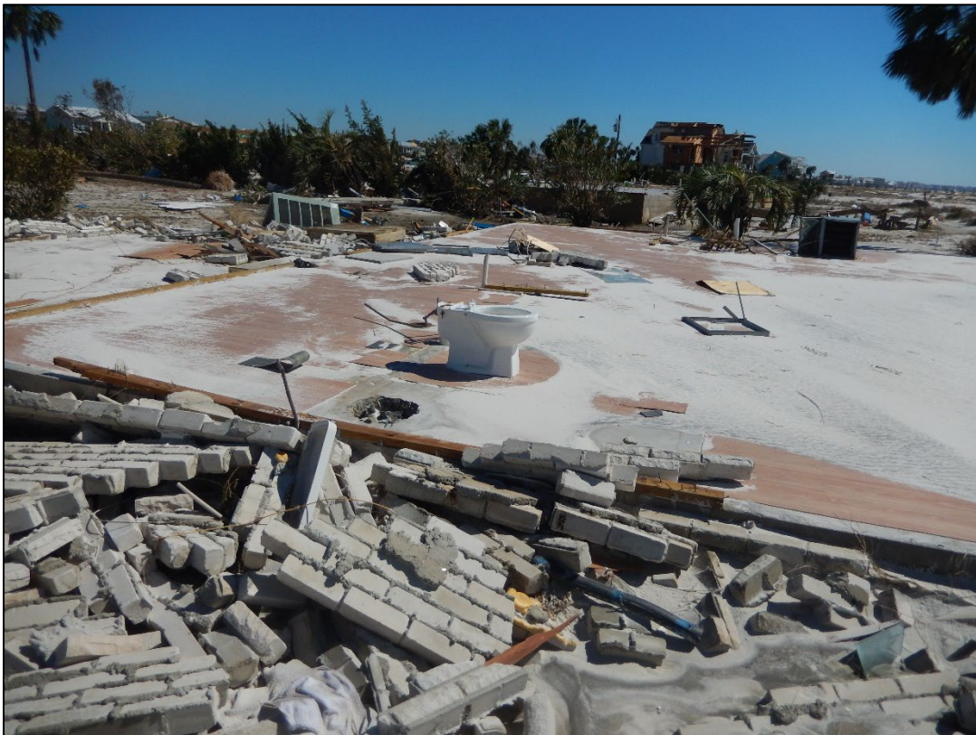
Figure 29. Remains of typical beach house destroyed near R128, Mexico Beach.
