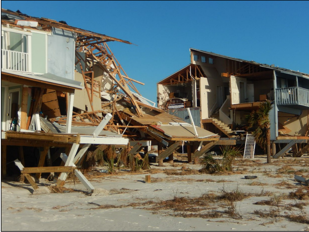
Figure 61. Townhouses destroyed near R7, Beacon Hill.
