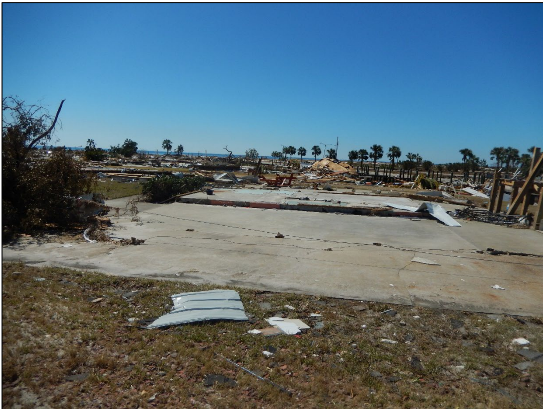
Figure 27. Rows of beach houses destroyed and removed by the storm surge, R127.5, Mexico Beach.
