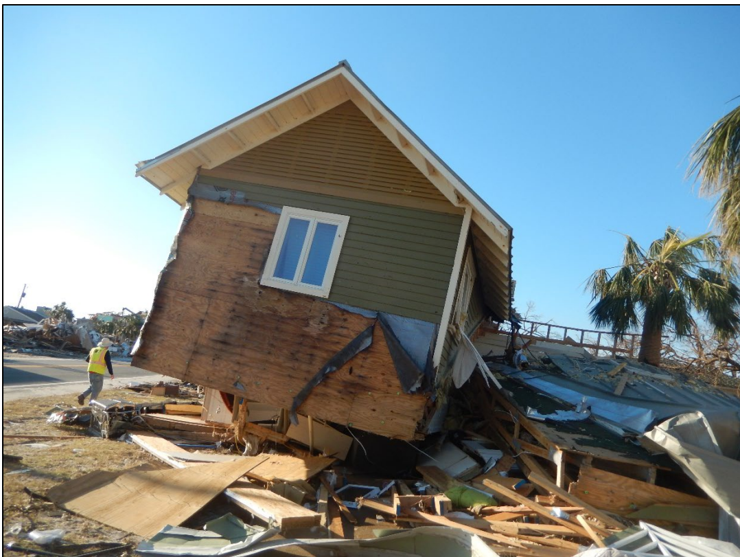
Figure 35. Beach dwelling transported across U.S. 98 by the storm surge, Mexico Beach.
