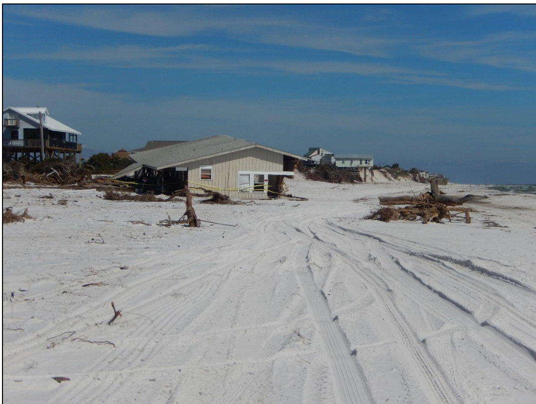
Figure 94. Dwelling destroyed near R174, Dog Island.
