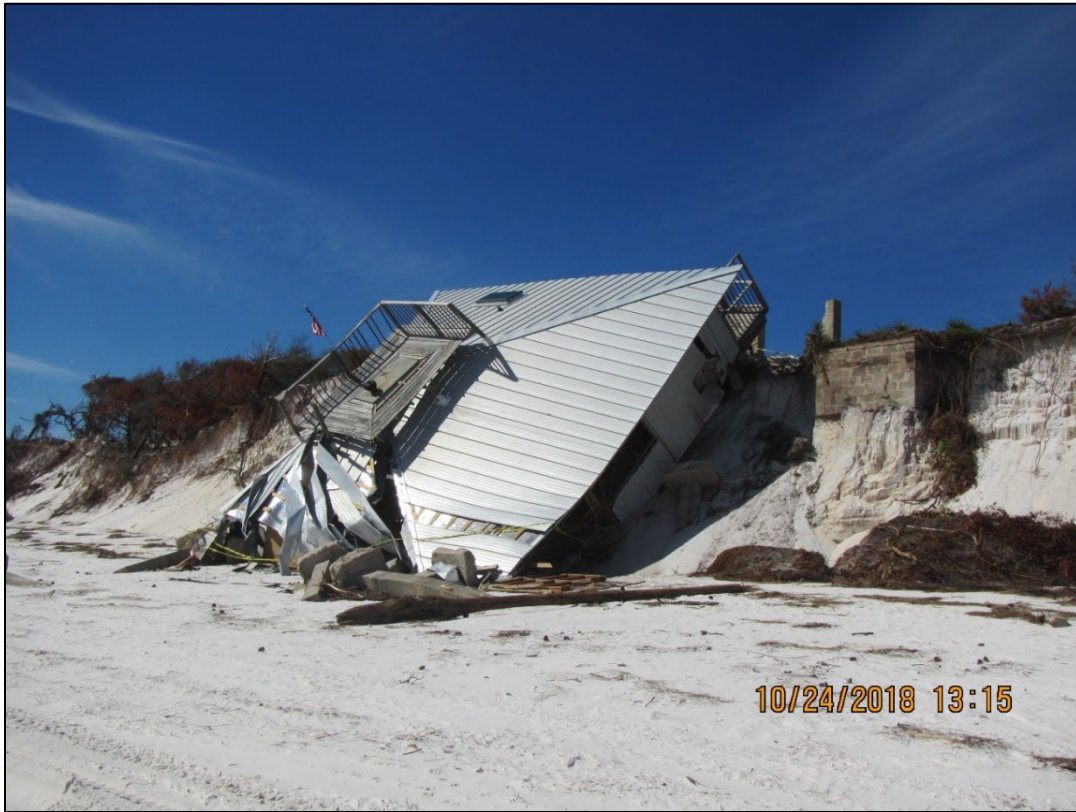
Figure 93. Dwelling destroyed near R173, Dog Island.
