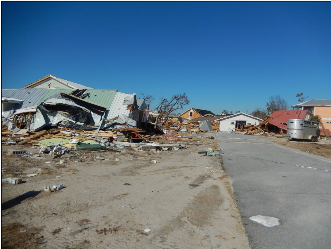
Figure 34. Buildings transported several hundred feet landward by the flood across U.S. 98 and deposited on 15 th Street, R130, Mexico Beach.
