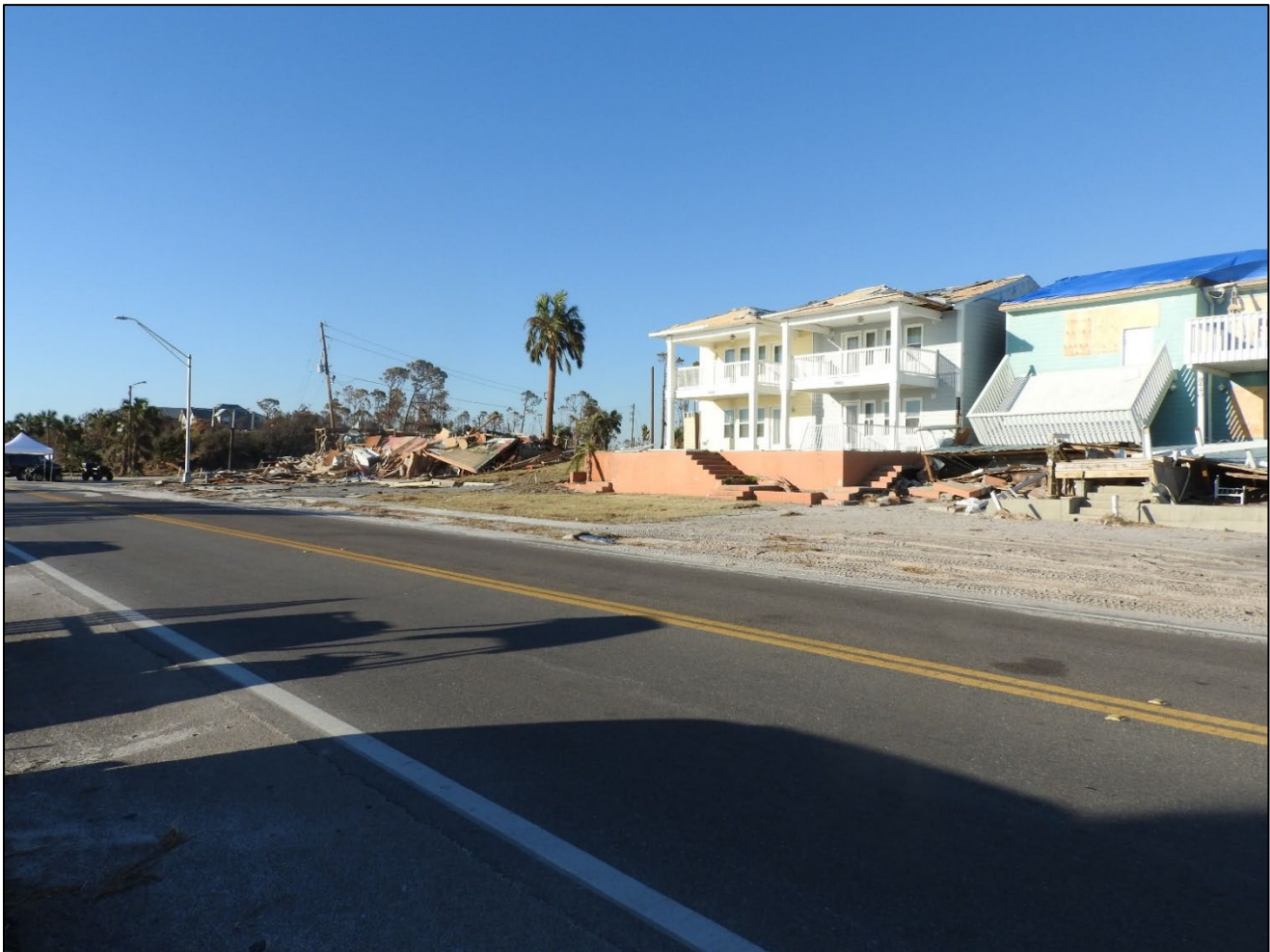
Figure 54. Site of high water mark of +21.2 feet NAVD along U.S. 98 and S.R. 386 near R1, Beacon Hill.
