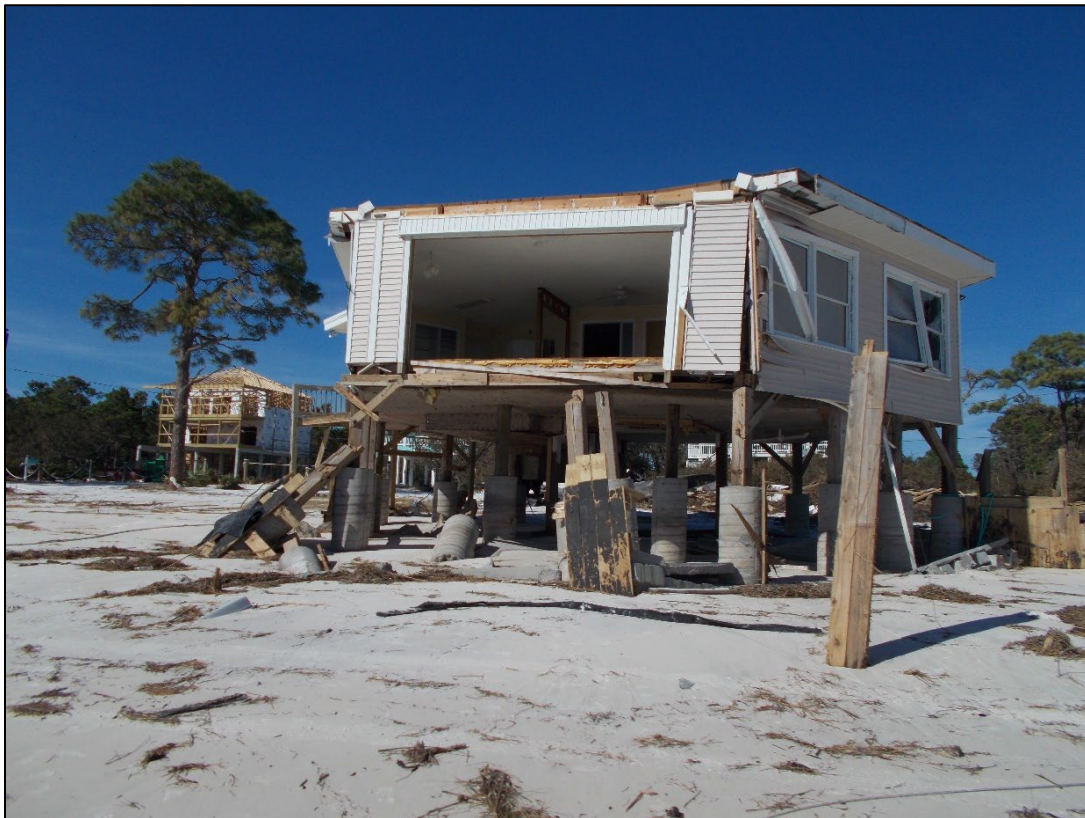
Figure 100. Dwelling destroyed near R210, Southwest Cape.
