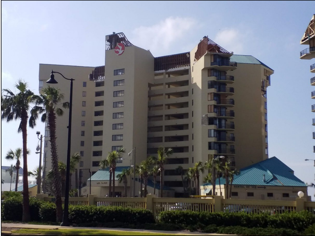
Figure 17. Wind damages on the Sunbird Condominiums near R67, Panama City Beach.
