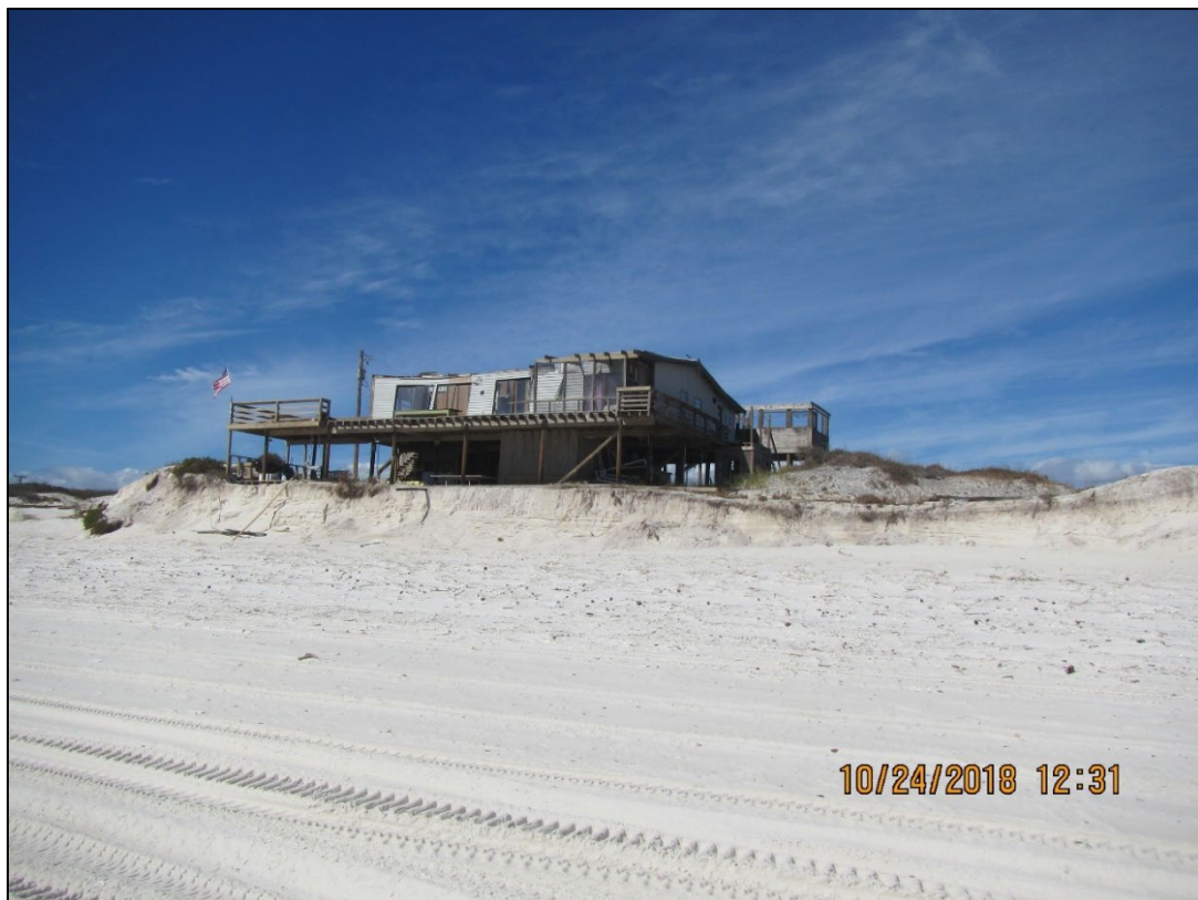
Figure 96. Dwelling destroyed near R178, Dog Island.
