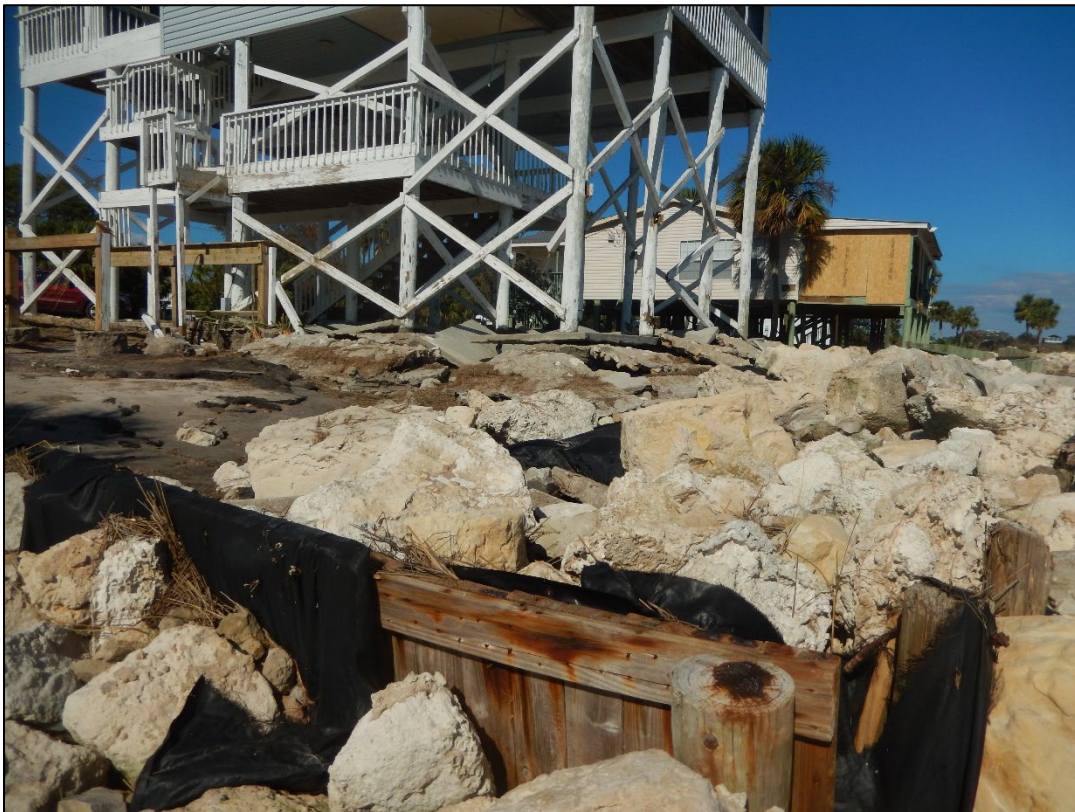
Figure 108. Rock revetment damaged and dwelling with parking slab and bracing damage at Shell Point, V361.
