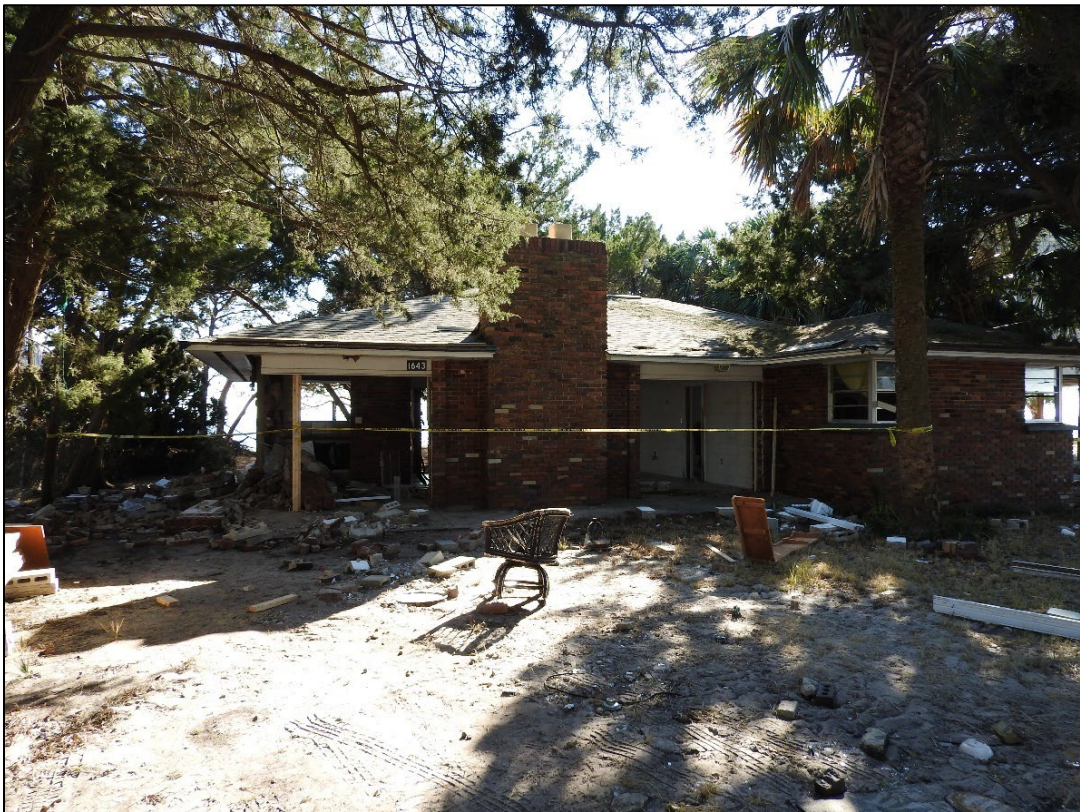
Figure 106. Dwelling with major damage from the storm surge at Shell Point, V342.
