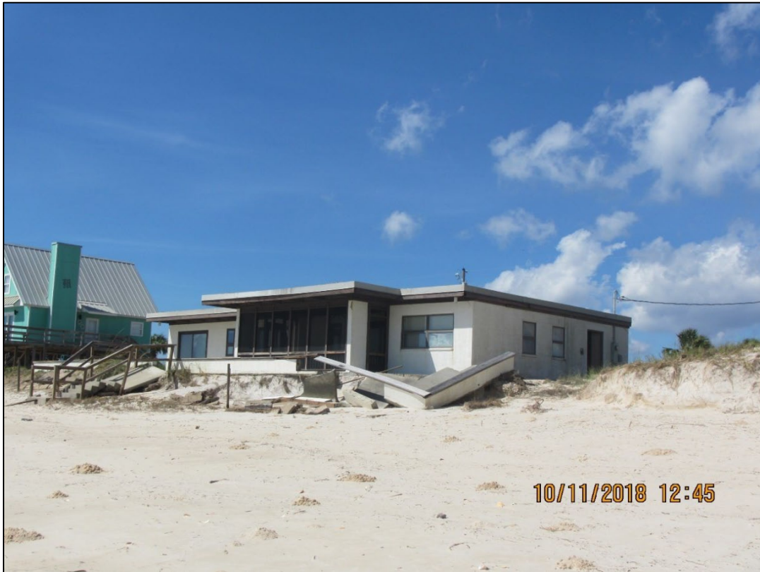
Figure 89. Dwelling damaged near R78, St. George Island.
