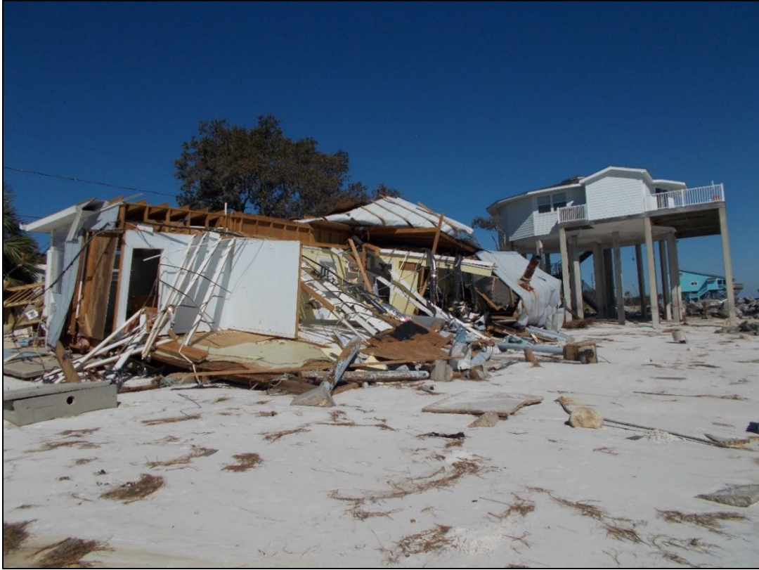
Figure 101. Dwelling destroyed near R211, Southwest Cape.
