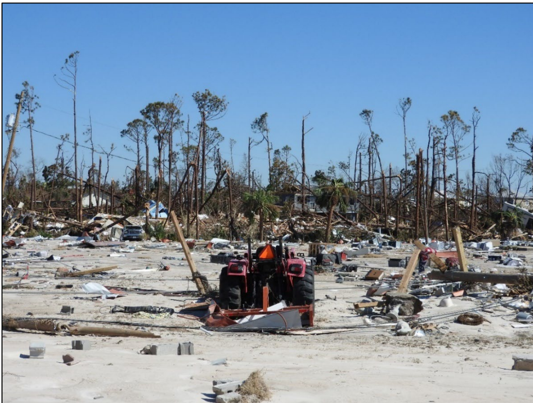
Figure 39. Storm surge transported debris and sand overwash across U.S. 98 near R135, Mexico Beach.
