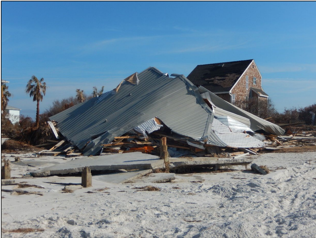
Figure 71. Dwelling destroyed near R99.5, St. Joseph Peninsula.
