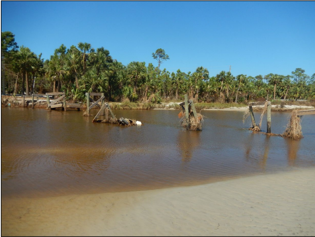
Figure 77. Bridge destroyed across Money Bayou, R140.5.
