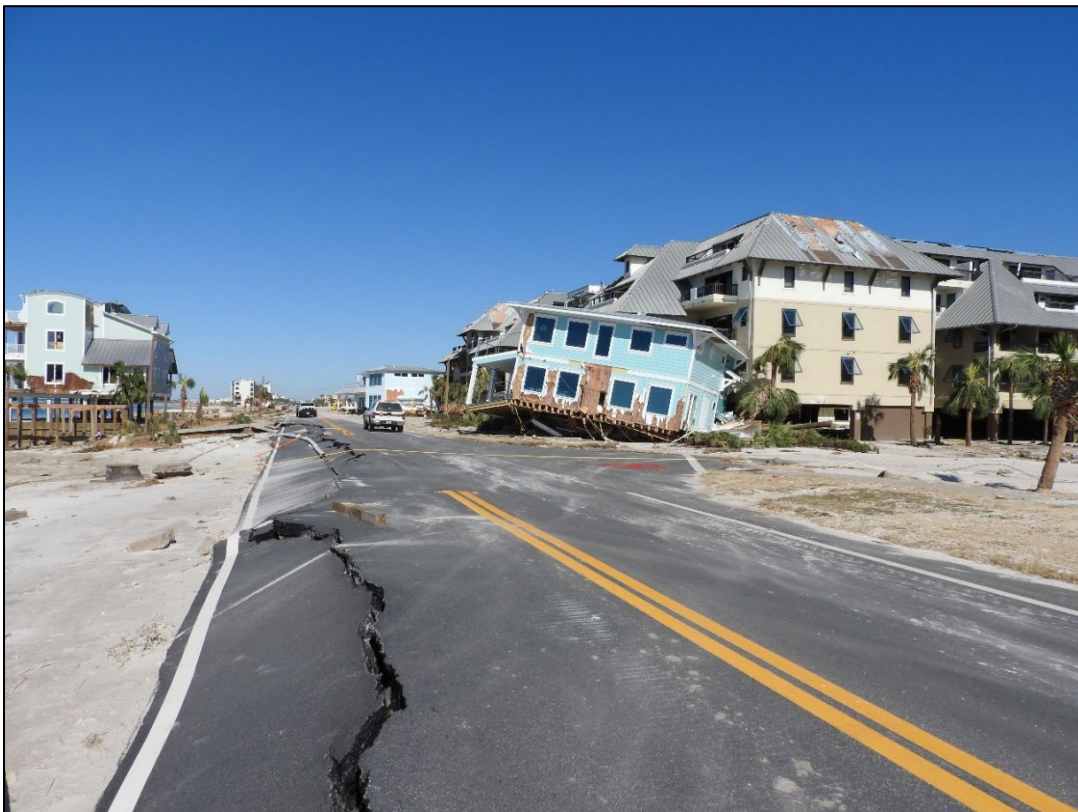
Figure 41. Dwelling transported across U.S. 98 by the storm surge near R136, Mexico Beach.
