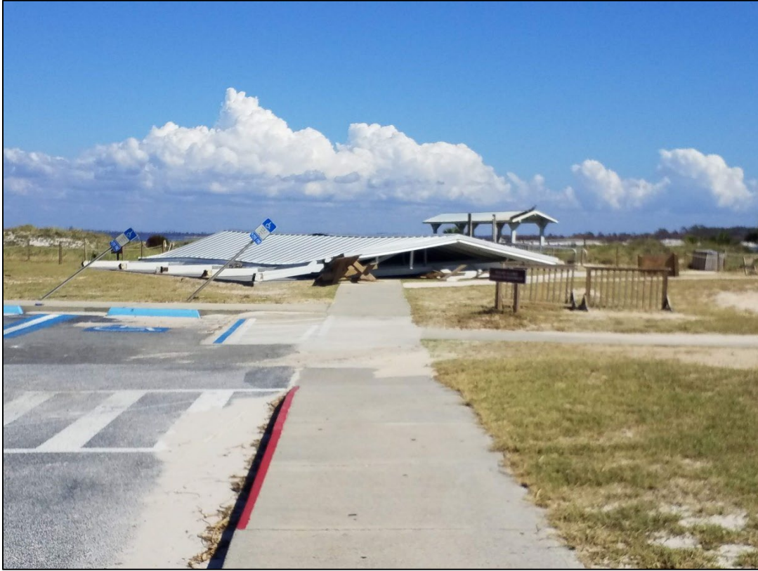
Figure 21. Collapsed pavilion near R97, St. Andrews State Park.
