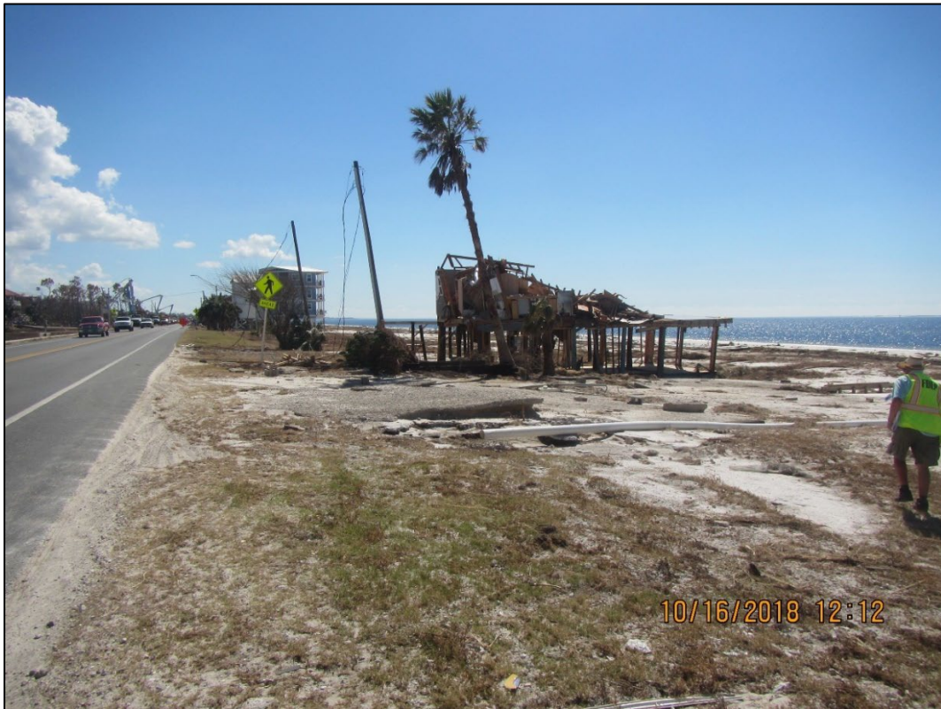
Figure 58. Dwellings destroyed along U.S. 98 near R3.5, Beacon Hill.
