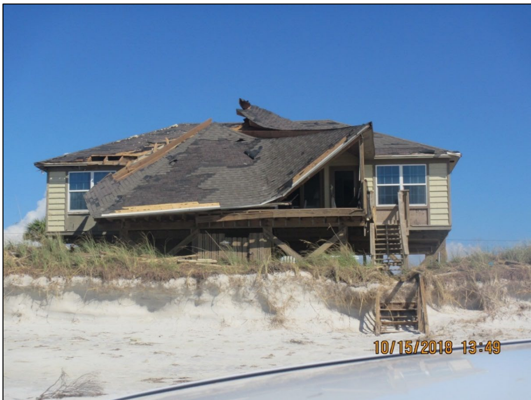
Figure 68. Major roof damage due to high winds near R85, St. Joseph Peninsula.
