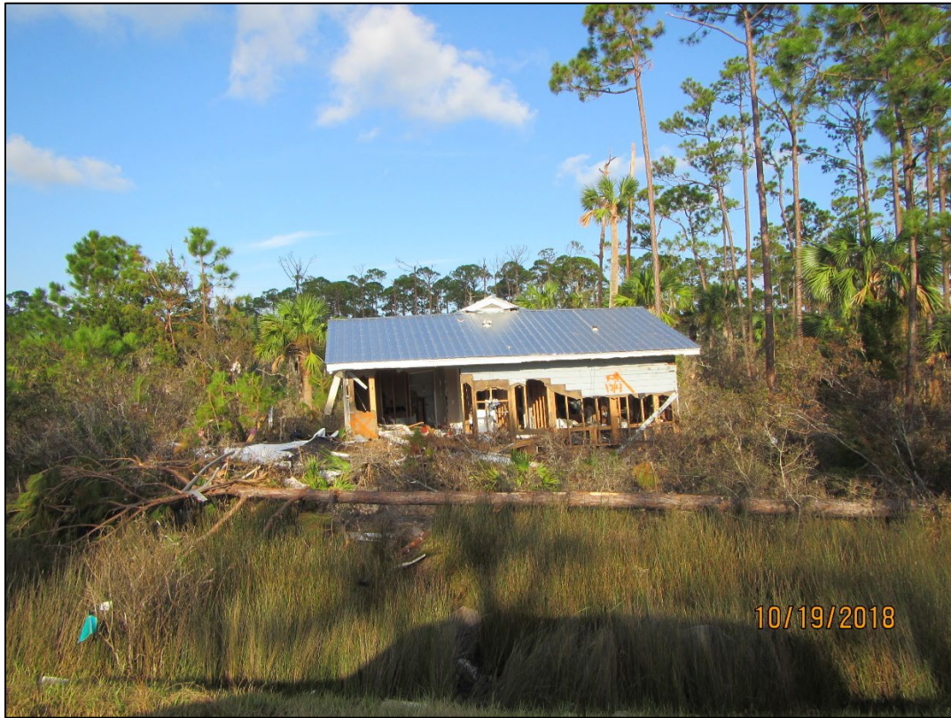
Figure 67. Destroyed dwelling transported across S.R.30A by the storm surge, St. Joseph Bay.
