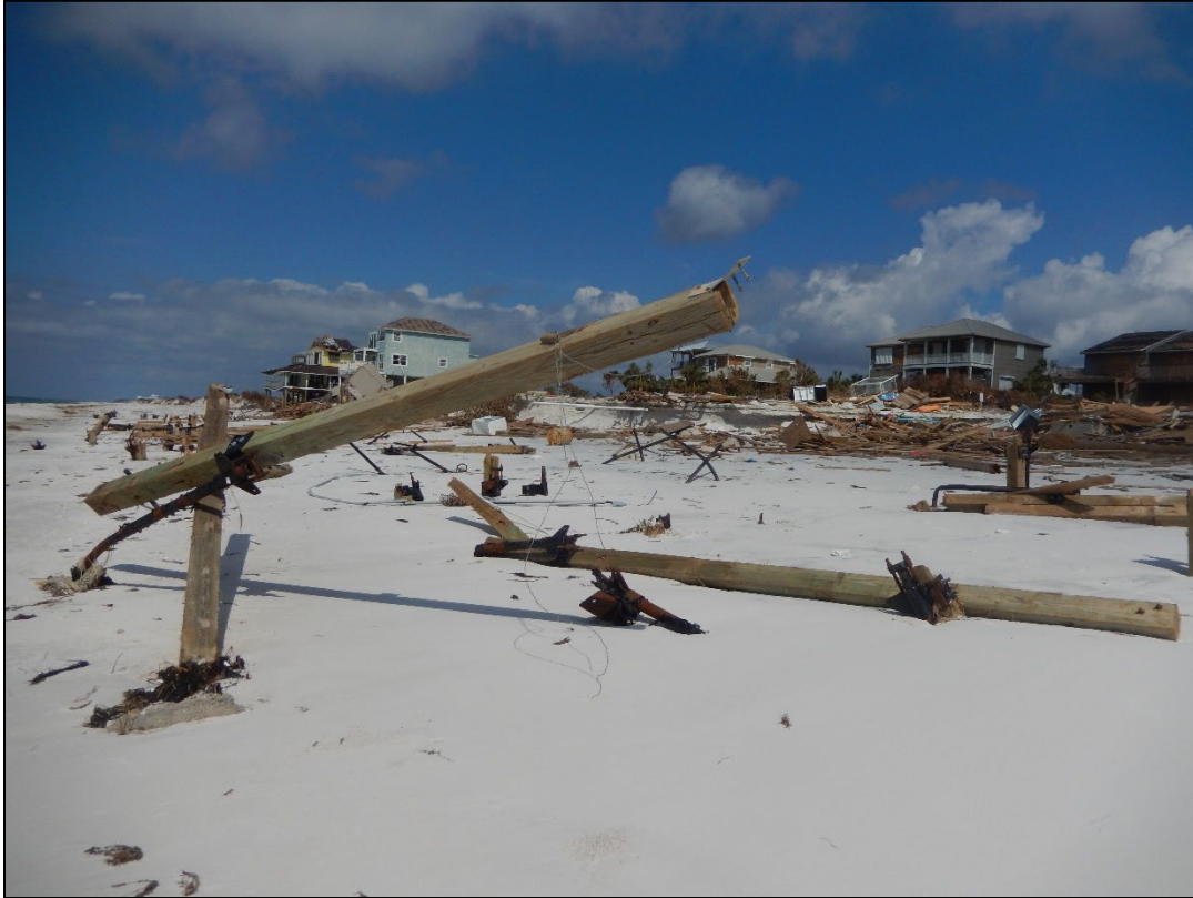
Figure 69. Remains of four destroyed townhouse buildings on Nassau Lane near R90.5, St. Joseph Peninsula.
