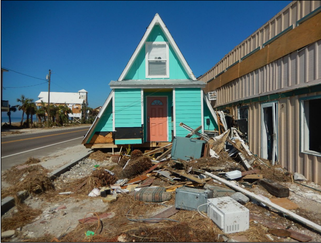
Figure 56. Dwelling transported across U.S. 98 by the storm surge near R2, Beacon Hill.
