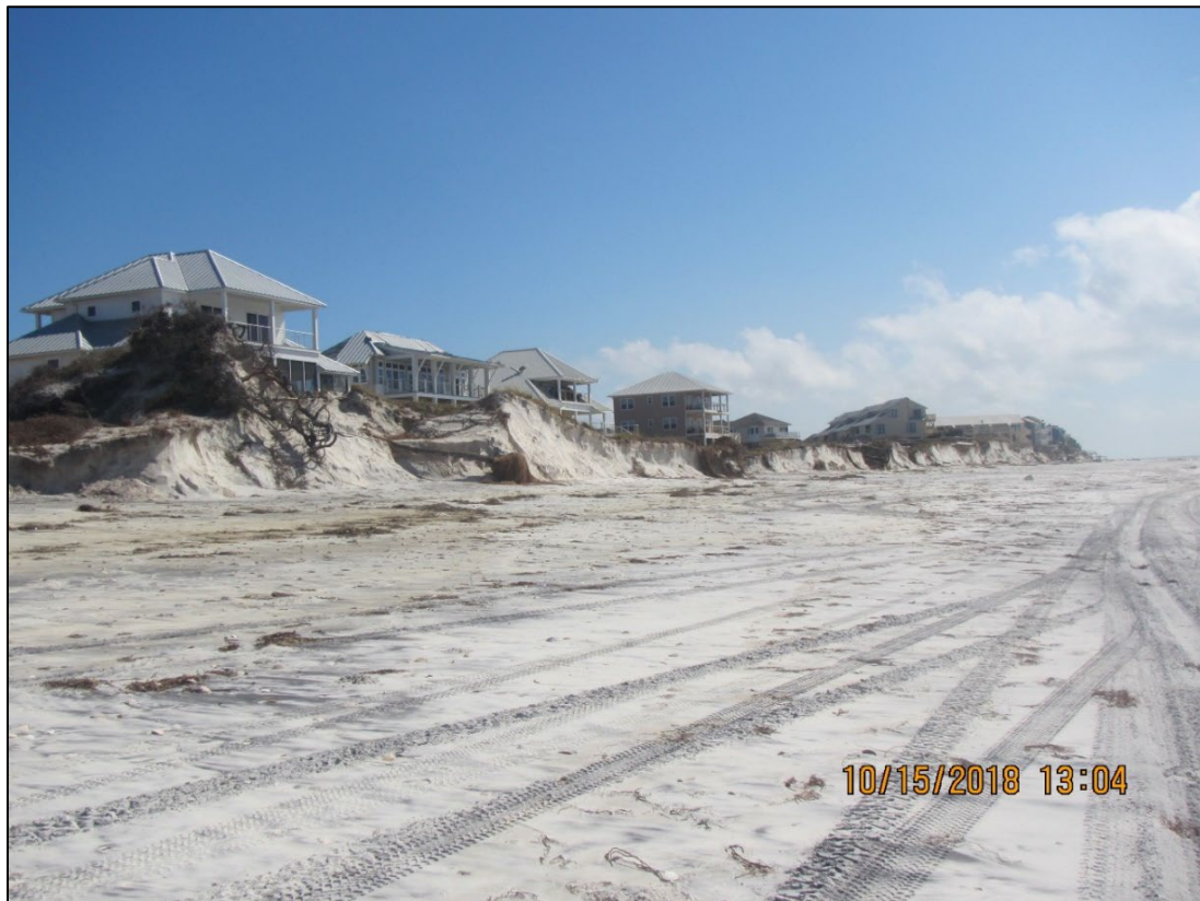
Figure 51. Major dune erosion, R77, St. Joseph Peninsula.
