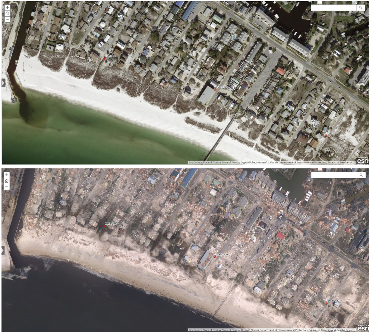
Figure 25. Aerial photo comparison of severe damage in Mexico Beach (R127.5-R130). Source: Vexcel Imaging/ NICB Geospatial Intelligence Center.
