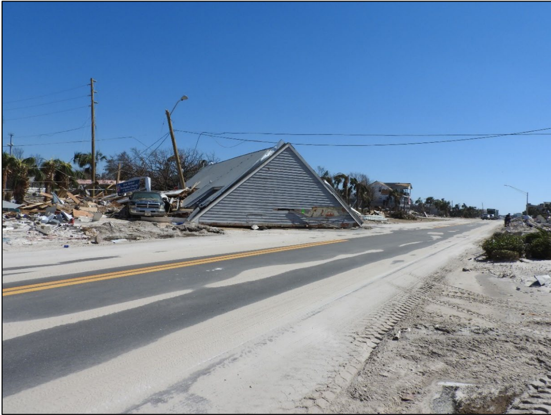
Figure 42. Roof of dwelling transported across U.S. 98 by the storm surge near R138, Mexico Beach.
