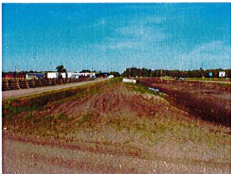
ROW improvements west of Hastings
