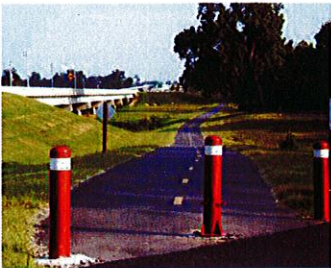
Bollards at a trail road crossing. The center bollard is removable to allow law enforcement and emergency vehicle access.
