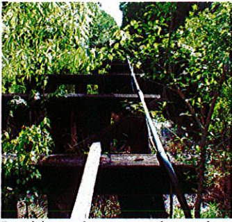
Remaining trestle structure at deep creek
