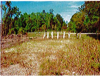
ROW crossing at SR207
