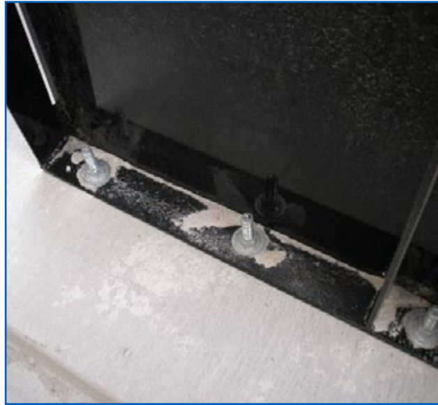
Check Tank Foundation and Anchoring
