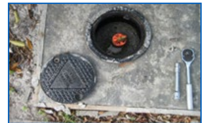
Cap in Place
