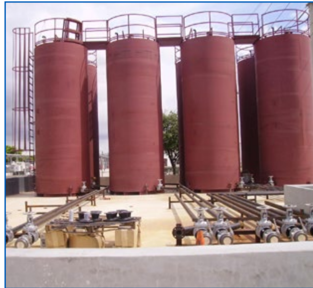
Check for Proper Secondary Containment Dimensions
