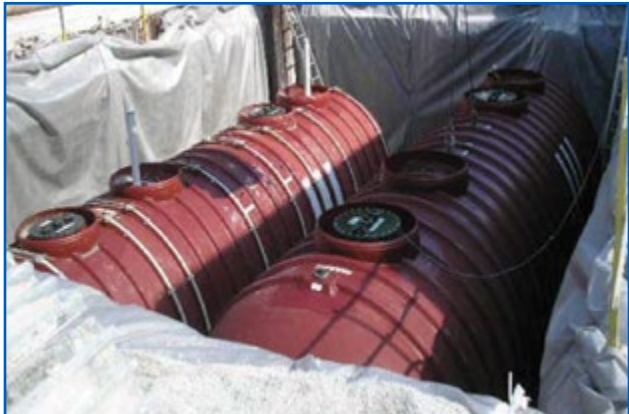
DW-Fiberglass USTs During Installation
