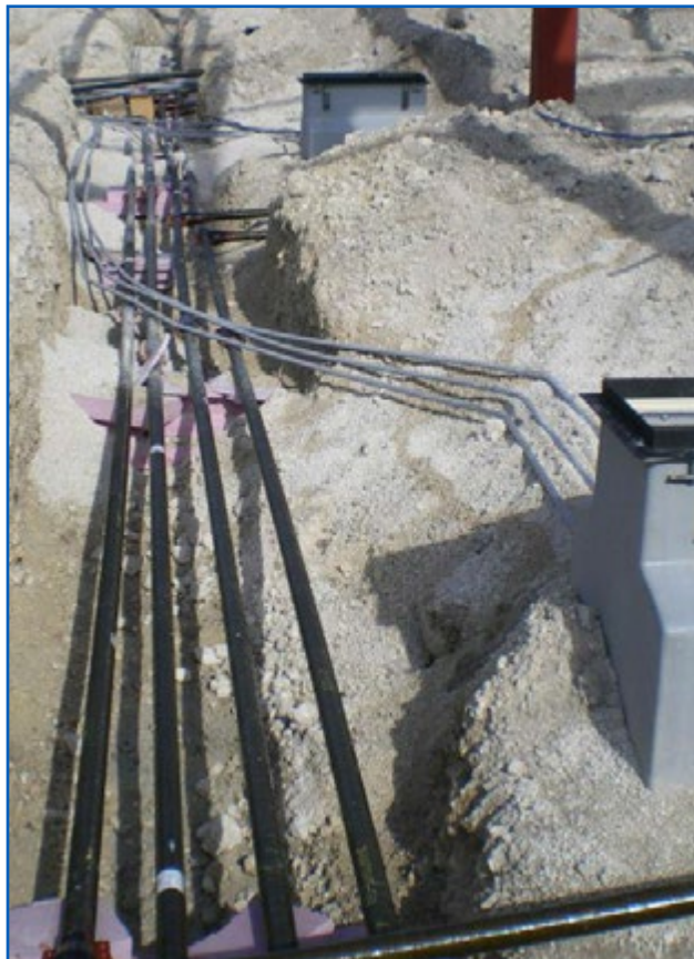
UST System Piping/Dispenser Liner Installation
