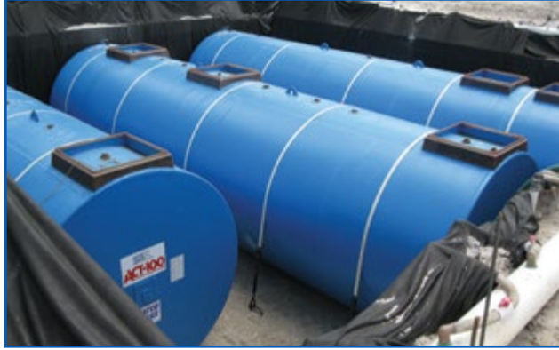
DW-Fiberglass Coated Steel Composite USTs During Installation
