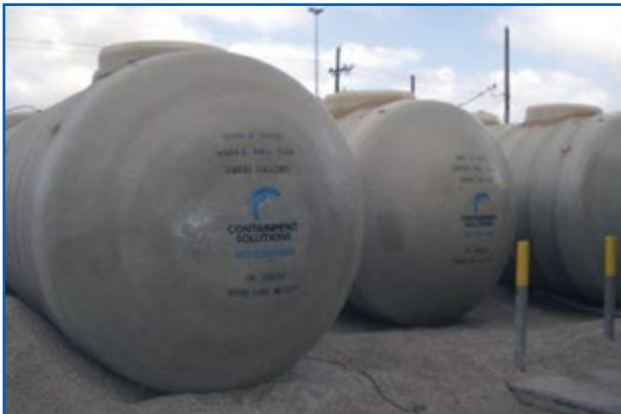
DW-Fiberglass USTs On-site, Pending Installation
