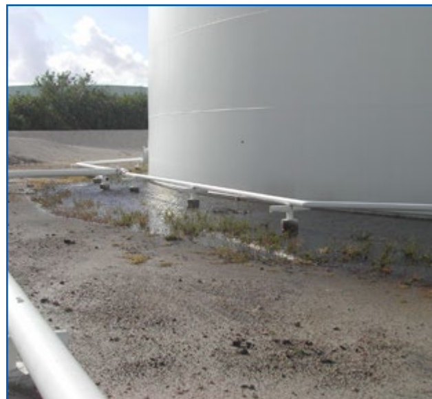
Check Secondary Containment for Discharge or Liquid Accumulation
