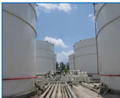
Piping for Field Erected AST
