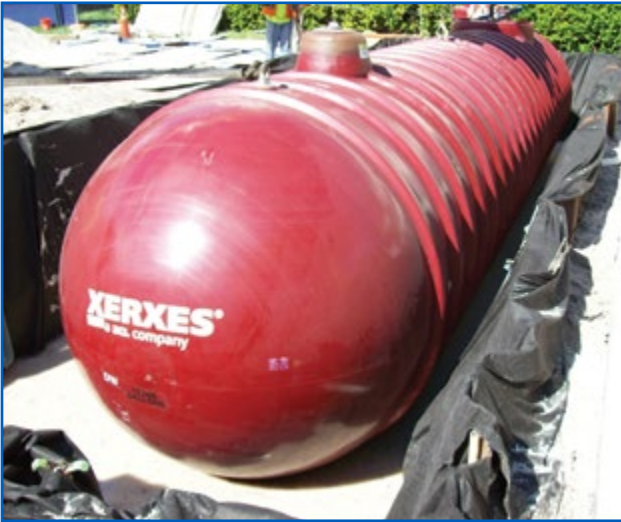
Double-walled Fiberglass UST with Brine-filled Interstice
