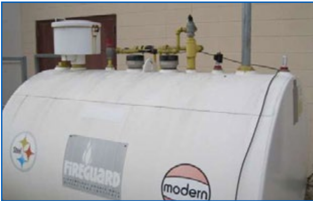
DW-AST with Spill Containment, Anti-siphon Valve and RD
