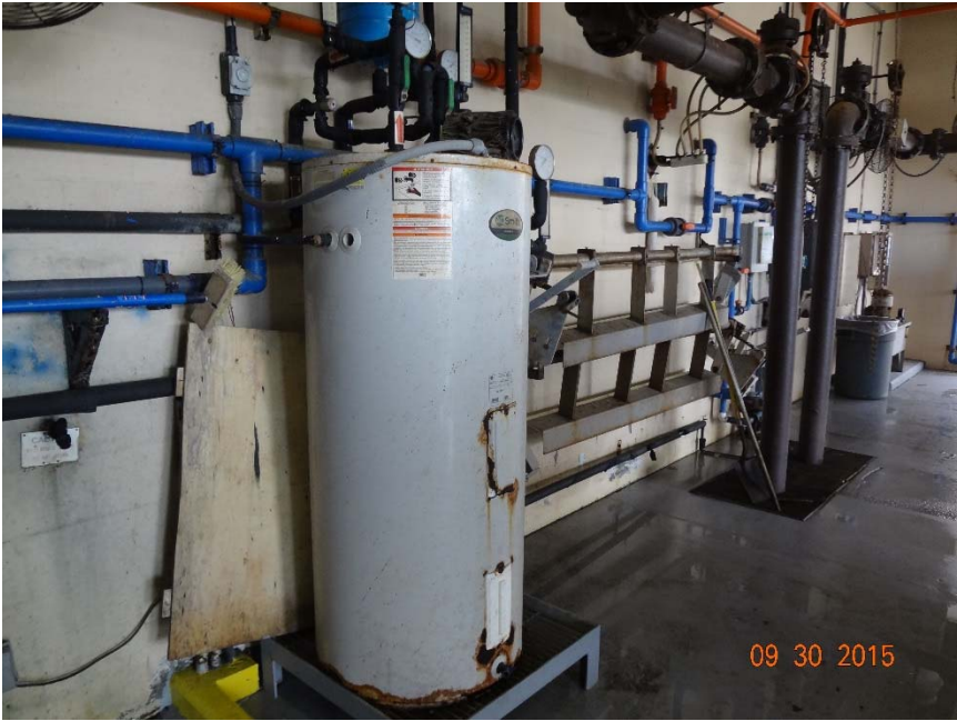
Figure NWWRF-2. Gravity Belt Thickener Piping Northwest WRF
