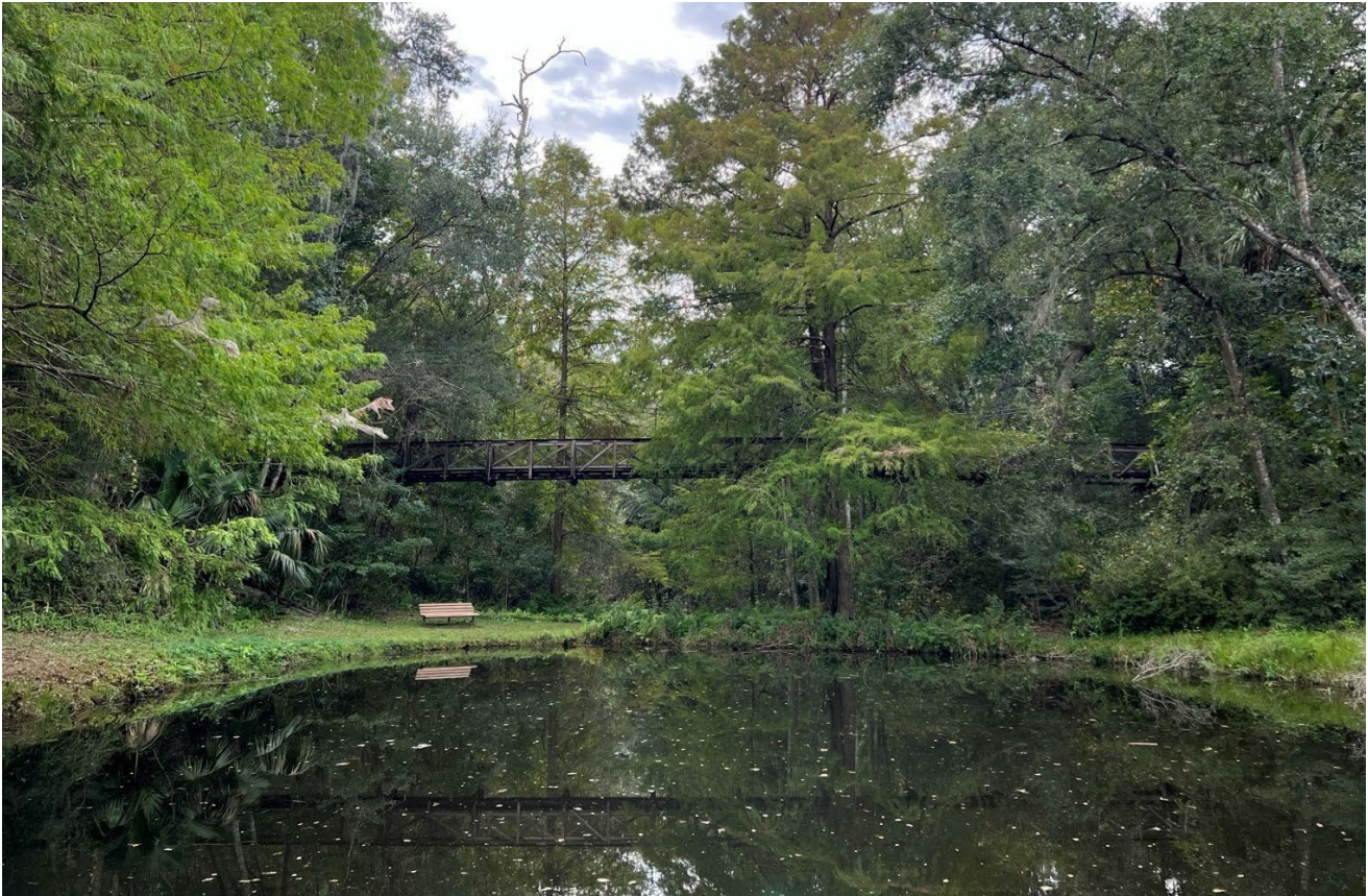
The Ravine: The 1934 suspension bridges found in the ravine area provide visitors a special way to observe the scenic features of this park. The two existing bridges were restored in 2005 but should be inspected for structural integrity again and repaired as necessary.
