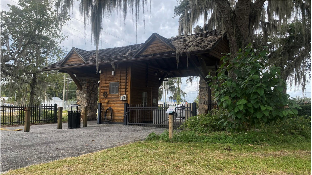
1934 Entrance Station: This historic and noteworthy feature of the park is no longer in use. Resuming some adaptive use of this entrance feature for park events and holidays would help ensure general upkeep and maintenance.
