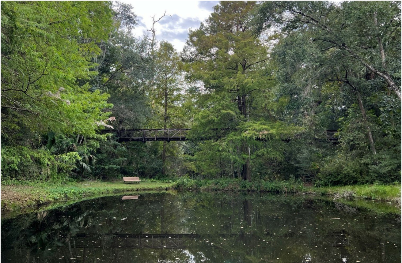
The Ravine: The 1934 suspension bridges found in the ravine area provide visitors a special way to observe the scenic features of this park. The two existing bridges were restored in 2005 but should be inspected for structural integrity again and repaired as necessary.
