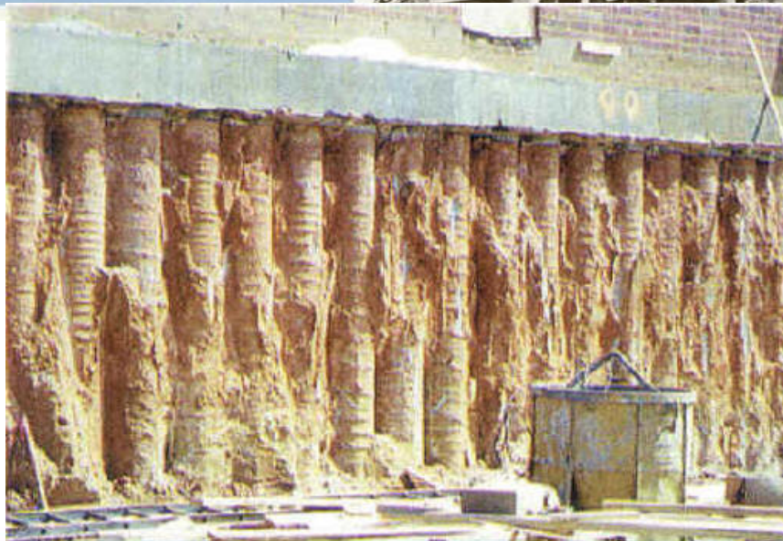
d) Water interrupt wall, grouting water-proof-chemicals
