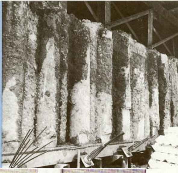
d) Water interrupt wall, grouting water-proof-chemicals
