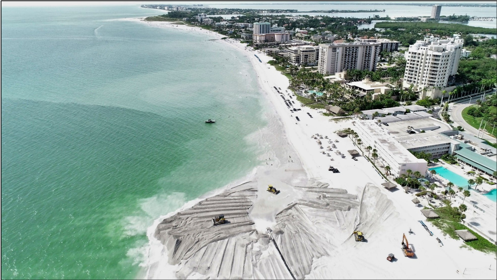
Lido Key Shore Protection Project being constructed in 2020 near R41. Photo courtesy of Camden Mill, P.E., with the City of Sarasota. See additional construction photos of beach nourishment projects.
