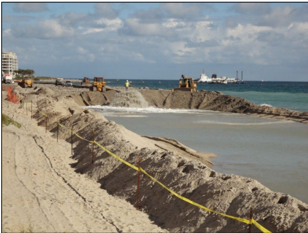
Figure 14. South Boca Raton beach nourishment project (2013) using sand from offshore sources. Photo courtesy of Peter Seidle, P.E.
