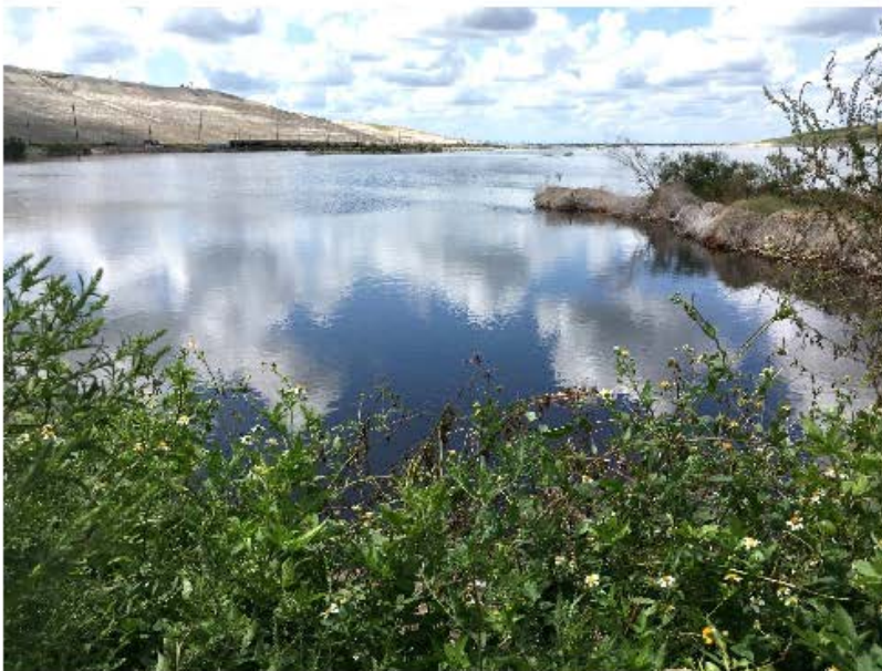
No. 10 Looking West over water-filled ditch- existing barrier. West end proposed fence here. (PS-19)
