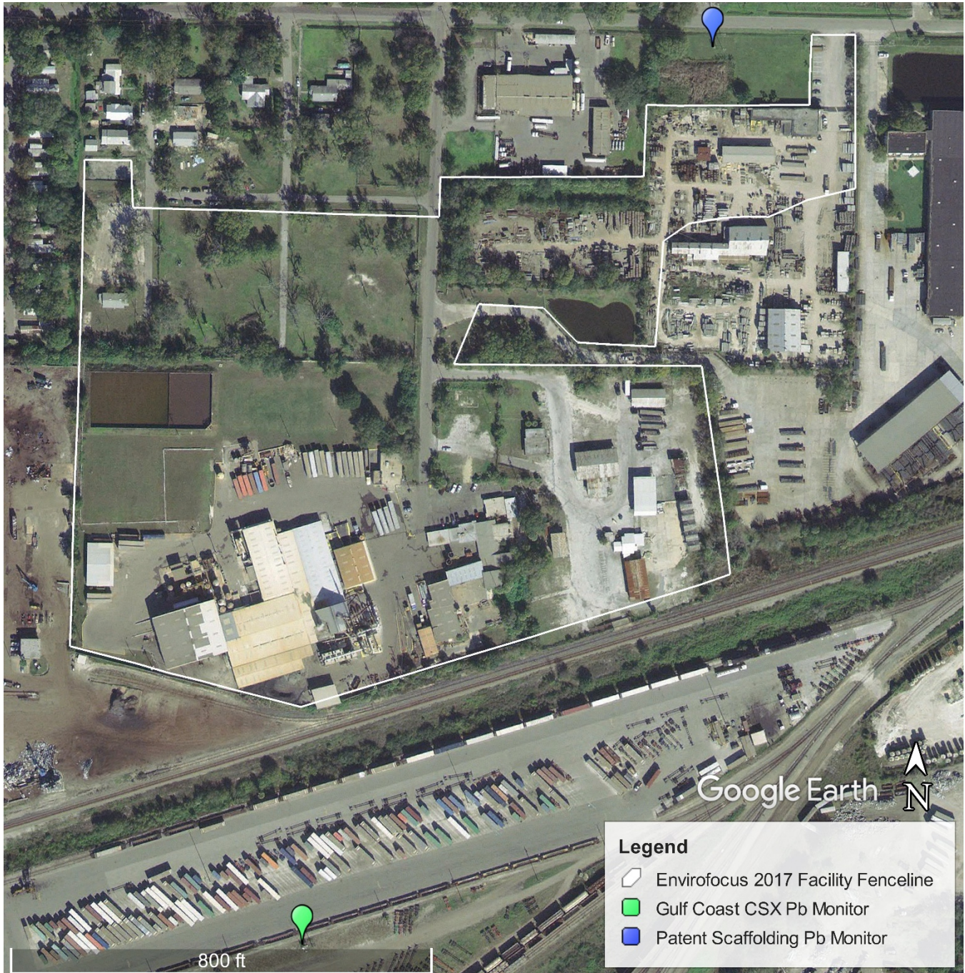
Figure 5: Satellite image of the Envirofocus facility before the reconstruction/modernization in 2007.
