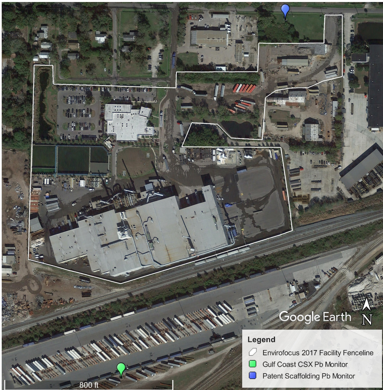
Figure 6: Satellite image of the Envirofocus facility after the reconstruction/modernization in 2017.
