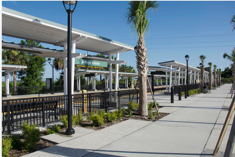
DeBary SunRail Station
