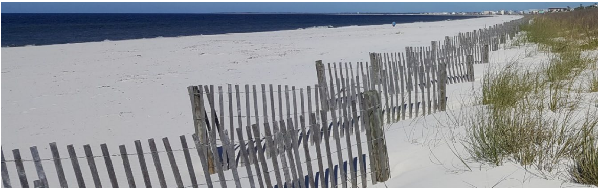
Figure 1: Sand fences installed to state of Florida specifications for the Mexico Beach dune restoration project built after Hurricane Michael. These sand collection fences have enlarged the new dune by trapping sand from the beach. Installation of sand fences in combination with planting vegetation has been a successful dune restoration method.
