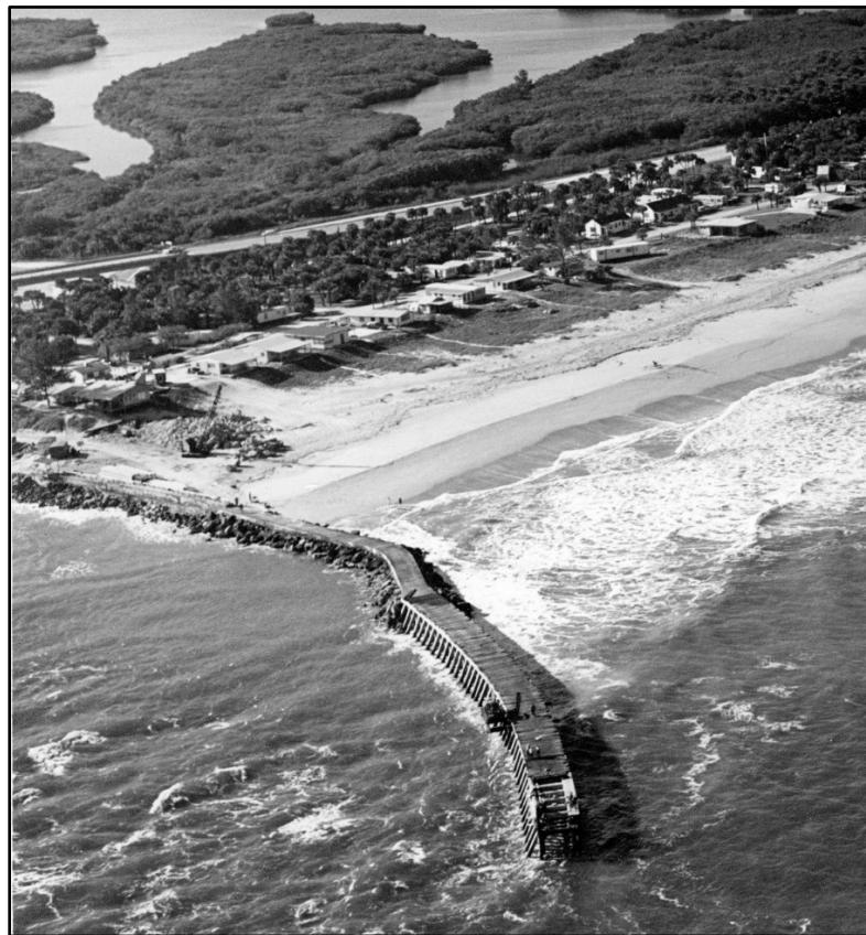
Figure 9. Extension of the north jetty at Sebastian Inlet, 1969, (Sebastian Inlet District, 2019).
