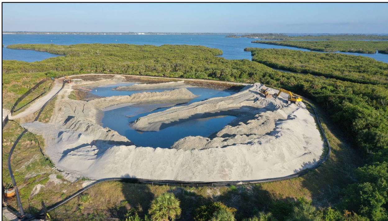
Figure 11. Dredge Material Management Area (DMMA) looking northwest, photo courtesy of Sebastian Inlet District.
