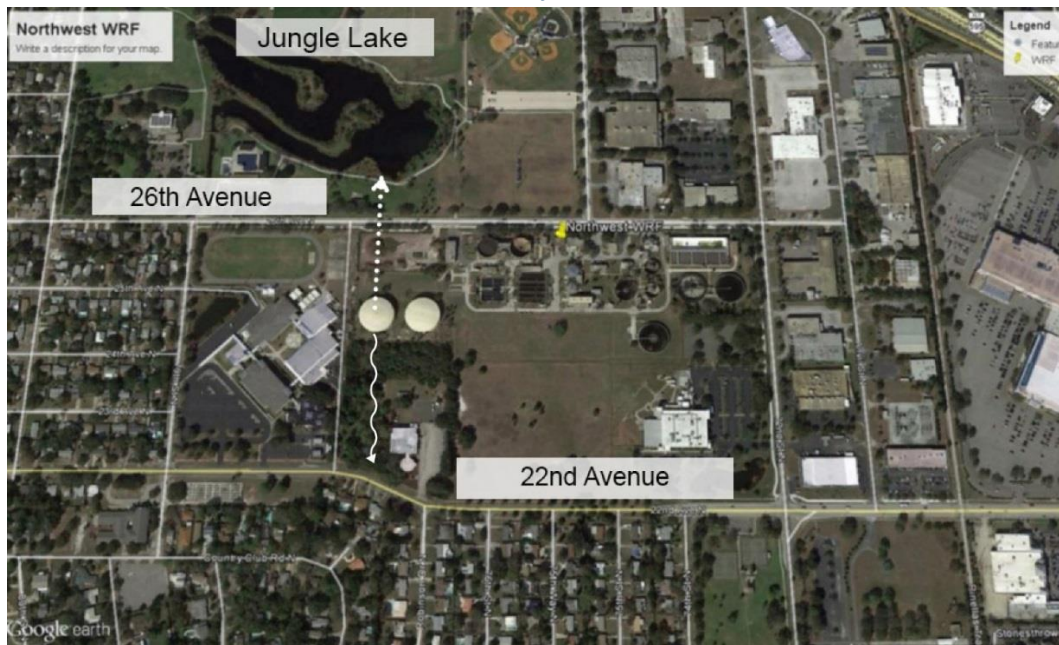
Figure 2. Locations of NWWRF reclaimed and reject water tanks overflow areas
