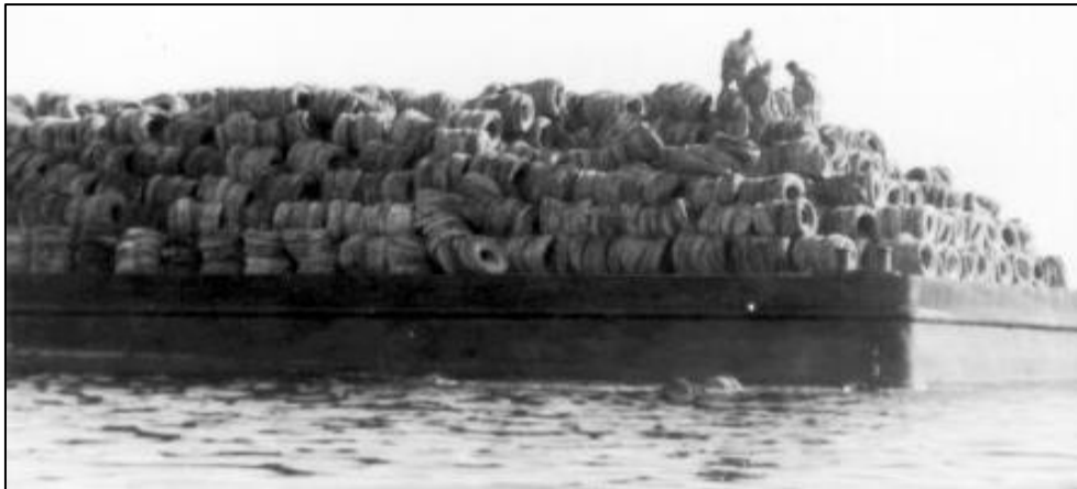
Image 1. Most of the tires deployed in the 1970s were placed as bundles.
