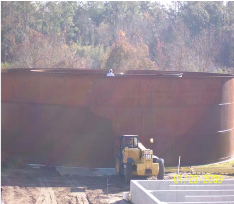
Figure 16: Digester #1/Clarifier #4 under construction
