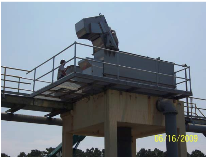
Figure 10: Mechanical barscreen assembly mounted on top of existing splitter box
