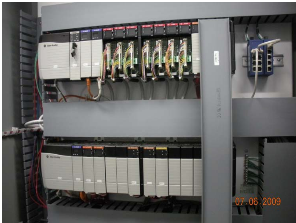
Figure 17: Programmable Logic Cards in MCC #5
