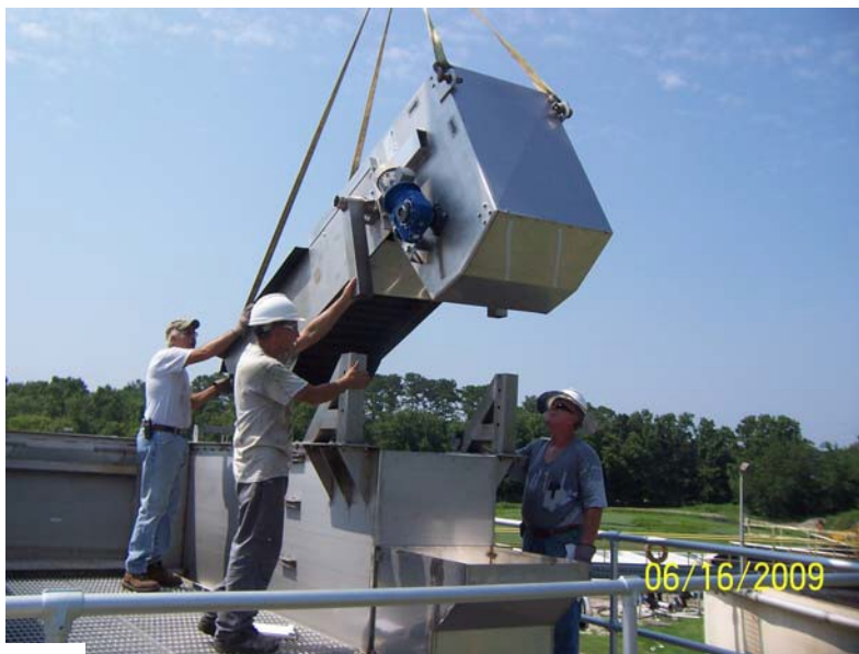
Figure 9: Installing Vanguard Mechanical barscreen in flow channel
