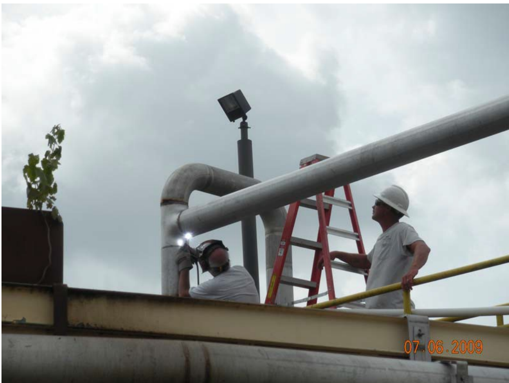
Figure 13: Connection of overhead air header to existing plant
