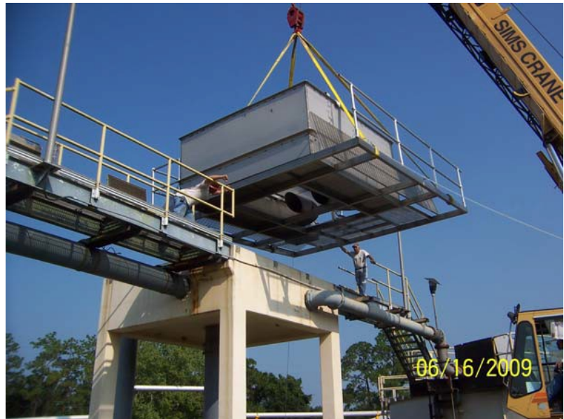
Figure 8: Hoisting Mechanical Barscreen channel into place atop the existing splitter box
