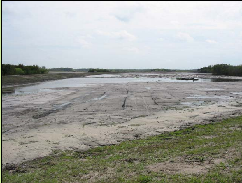
Recently constructed wetland, showing NO topographic relief (MTB).
