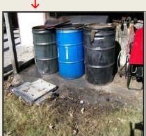
**♦ Secondary Containment:** 110% of the volume of the <u>largest</u> container or single-walled tank in an outside area.
