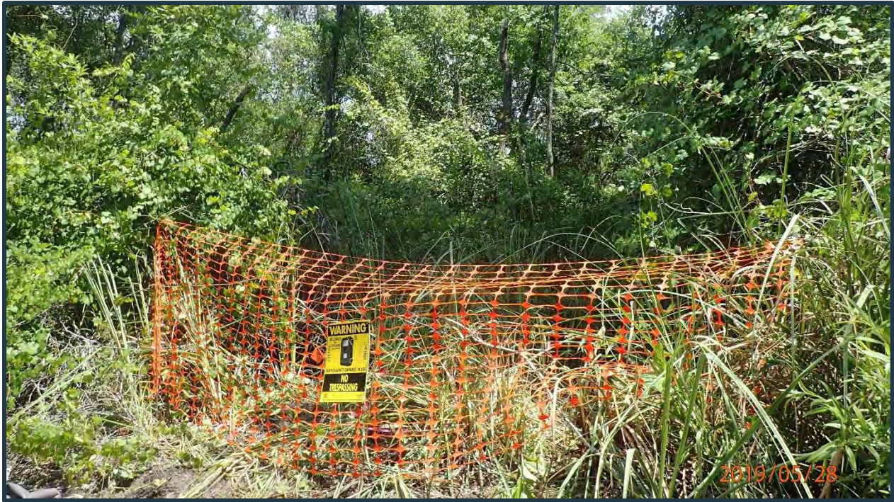
Figure 4.4 – Construction Fence Barrier
