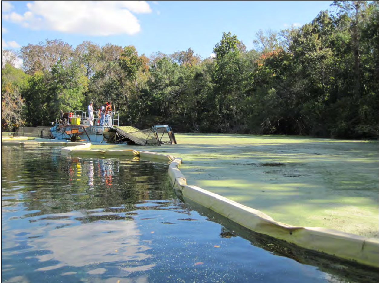
Hydrilla was mechanically removed from Wekiwa Lagoon after treatment with herbicide. Water flow is slowed by the turbidity barrier to improve the effectiveness of herbicide treatments.
