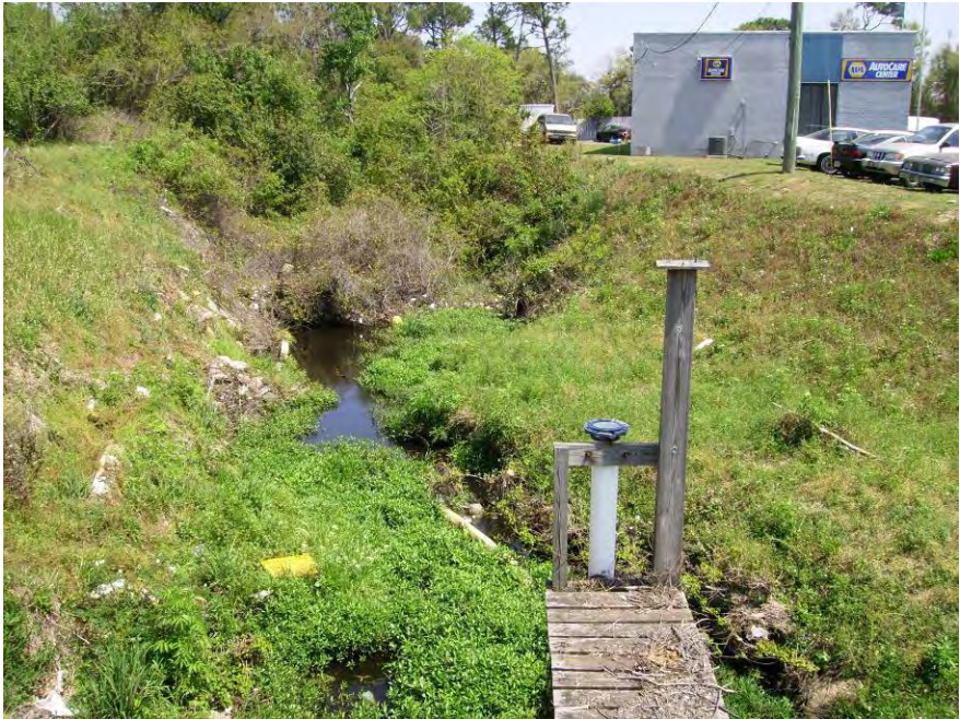
Jones Creek at North Navy Boulevard, downstream
