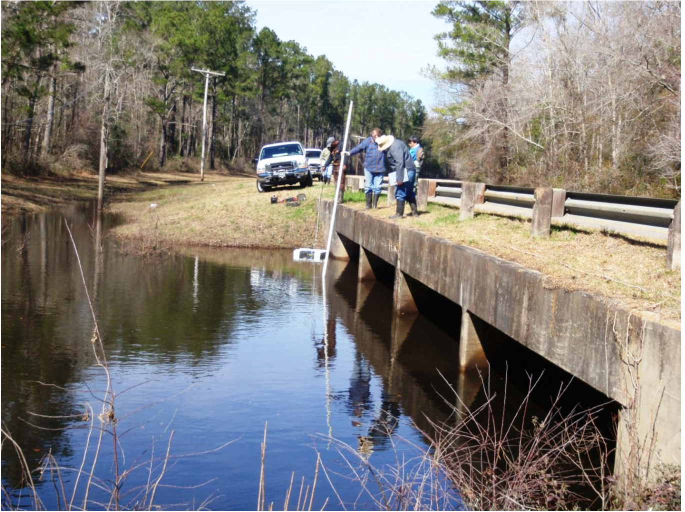
Figure 2.2. Most downstream station, PN0114 (R1), February 2010
