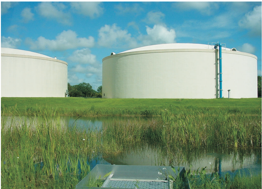
Water storage tanks at the Peace River Regional Water Treatment Plant in DeSoto County.
