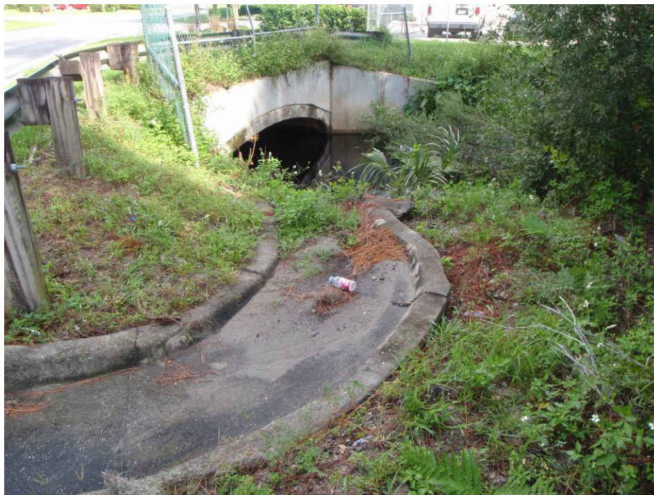
Figure 5.5. Stormwater Drain Flowing into Smith Canal at Station 21FLCEN 20010638
