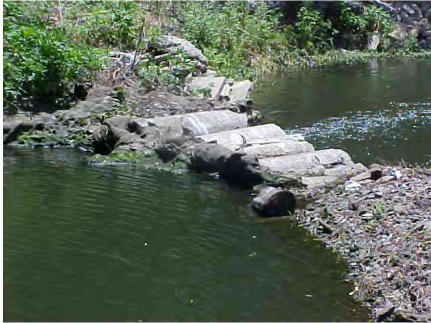
Figure H-1: Munson Slough near culverts upstream Lake Munson on 5-20-2008
