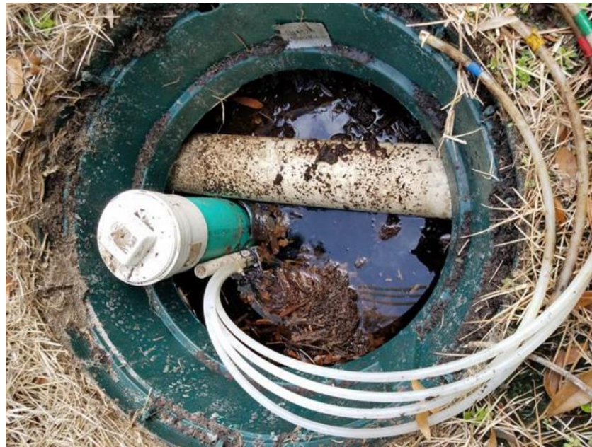
Lignocellulose Chamber when System BHS5 continued monitoring started in 2017
