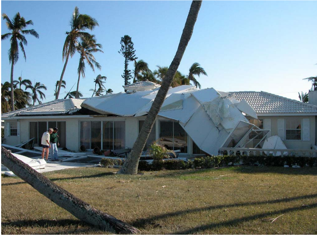
Photo 14. Damaged screen enclosure, south Naples (R86.9).
