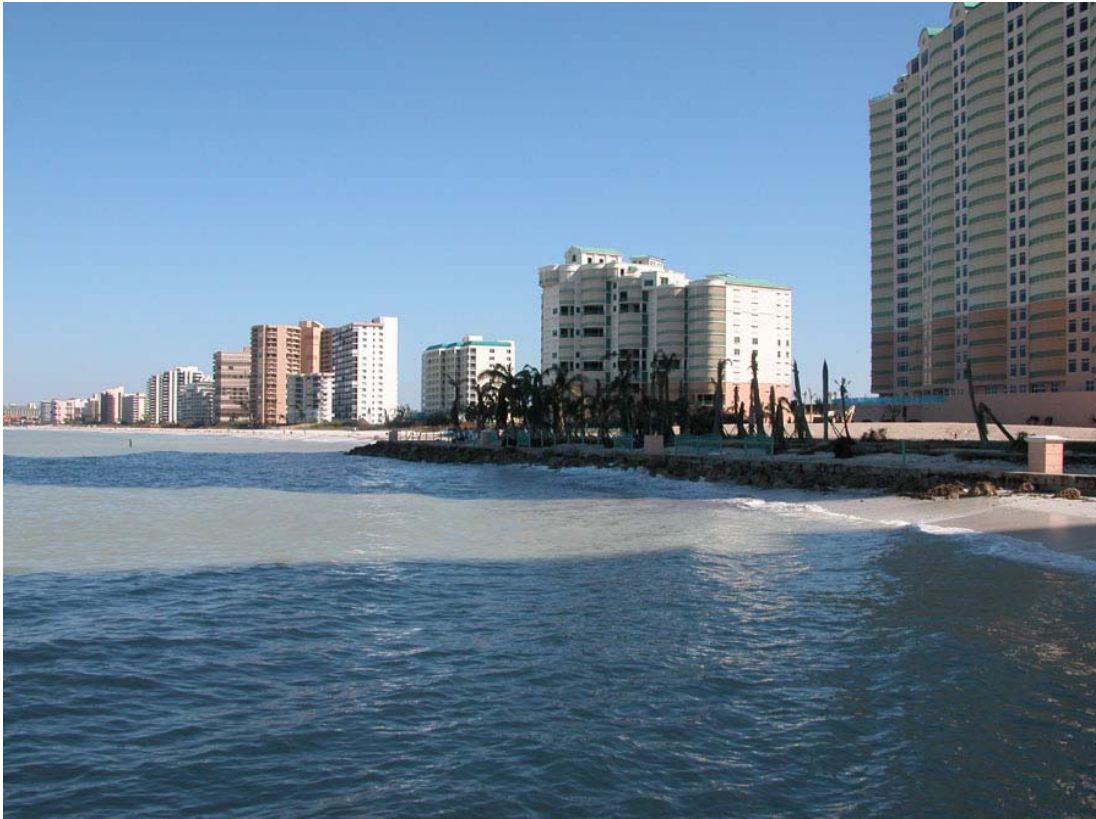
Photo 9. South Marco Island beach erosion (R148).
