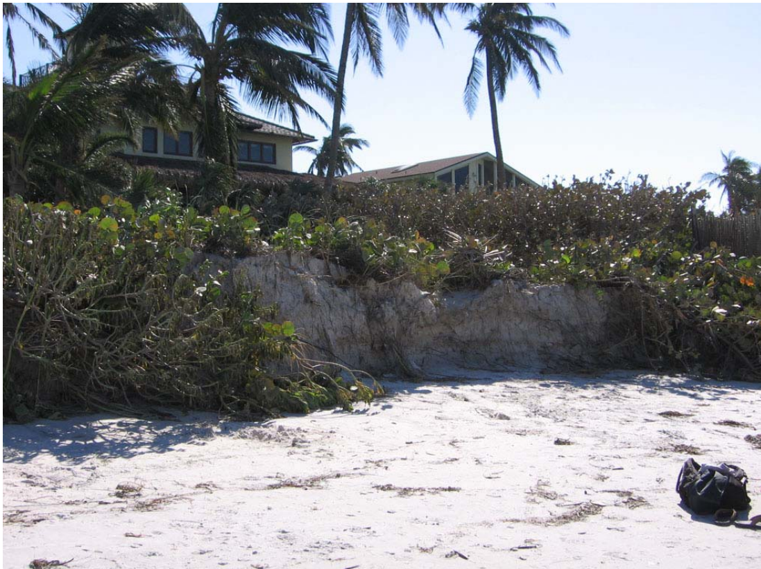
Photo 2. Moderate beach and dune erosion south of Naples Pier.
