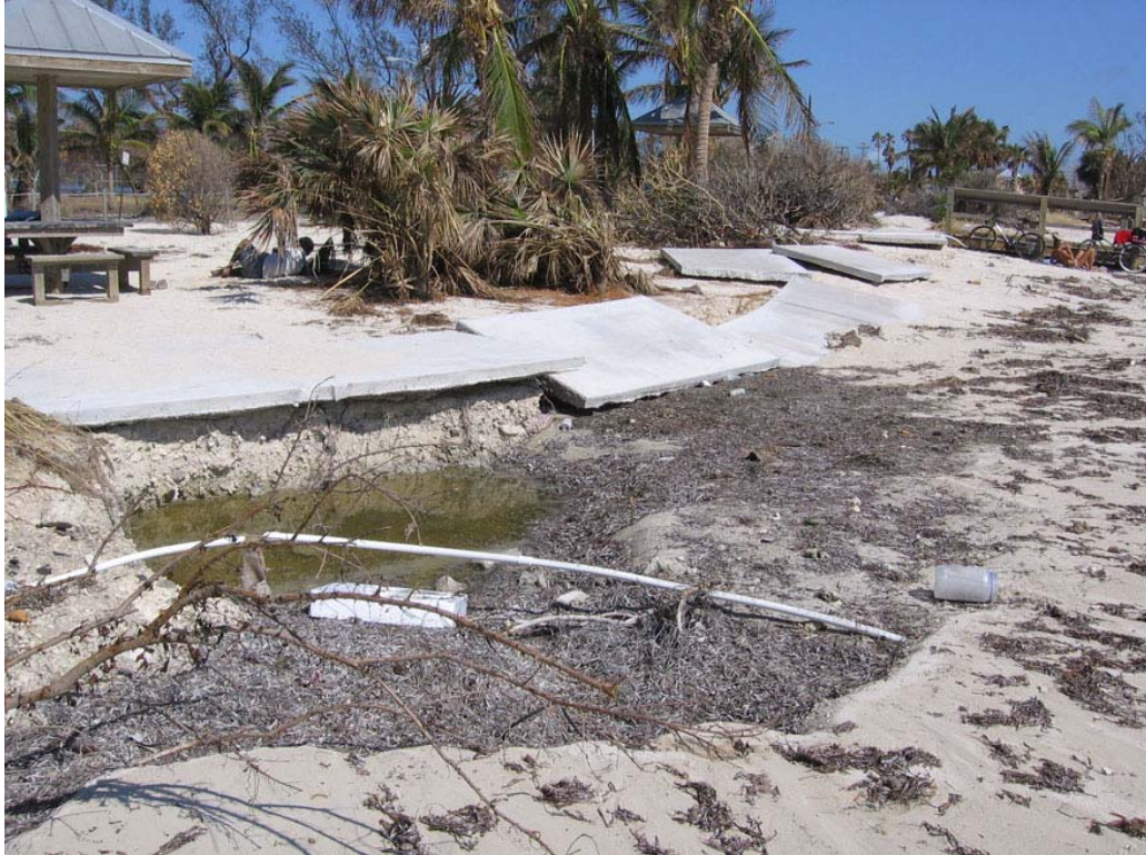
Photo 57. Damage to Rest Beach infrastructure.
