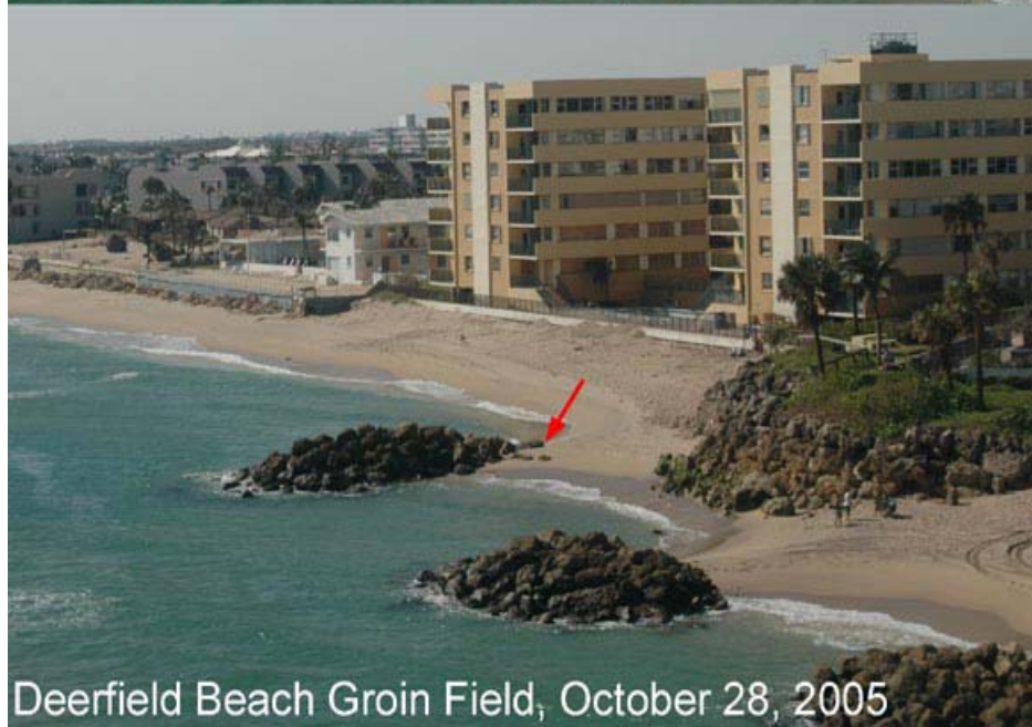
Photo 63. Moderate erosion at Deerfield Beach (R6.8).
