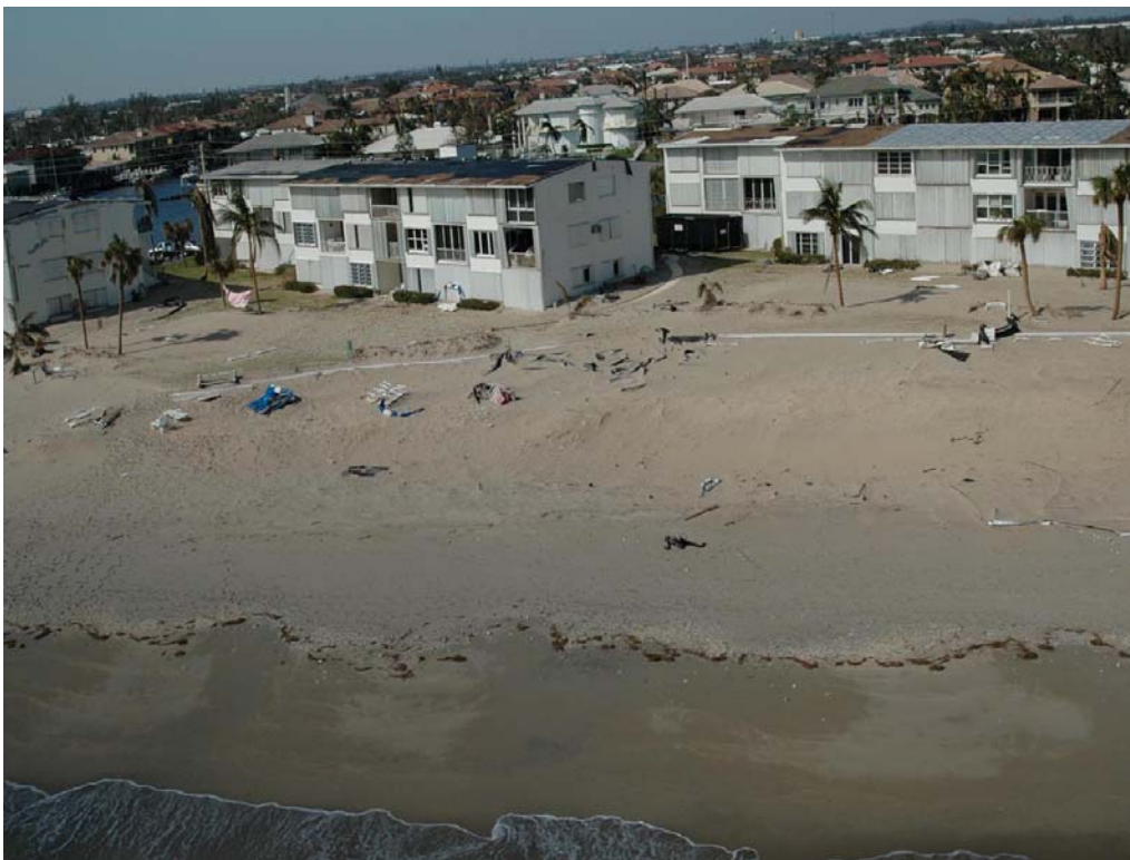
Photo 67. Damaged multifamily dwellings, Hillsboro Beach (R16.7)
